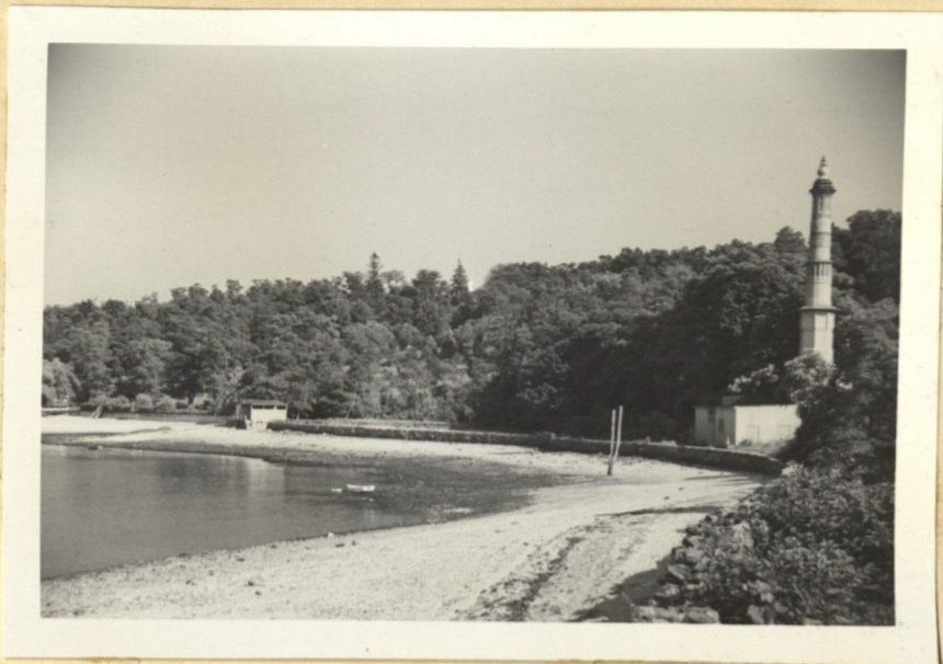
Side beach. Bath house & Power house. (Looking south.)
