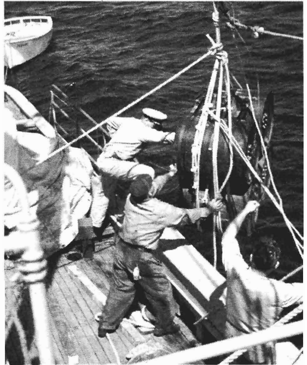
Assembled charge ready to hoist over the side, August 1949.
