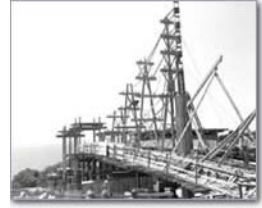
Construction of the Scripps Crossing bridge
