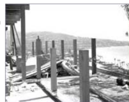
Support pillars for the Revelle Lab Building 3000
