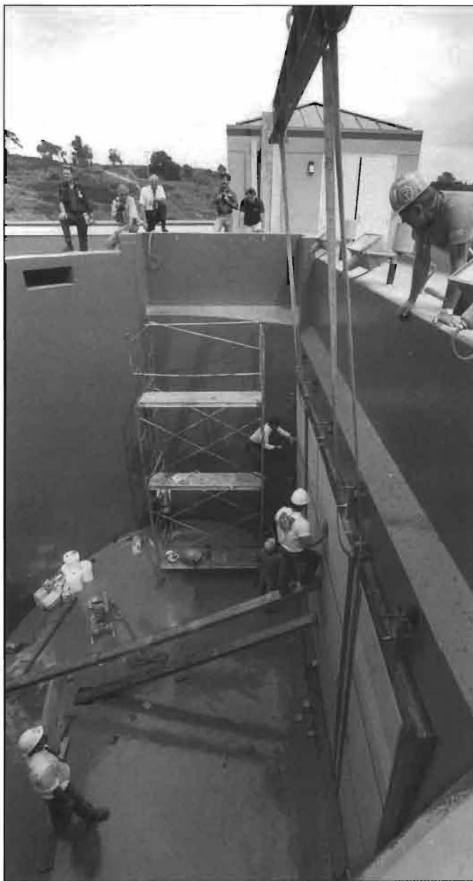
Workers seal the large acrylic window for the kelp forest exhibit.
