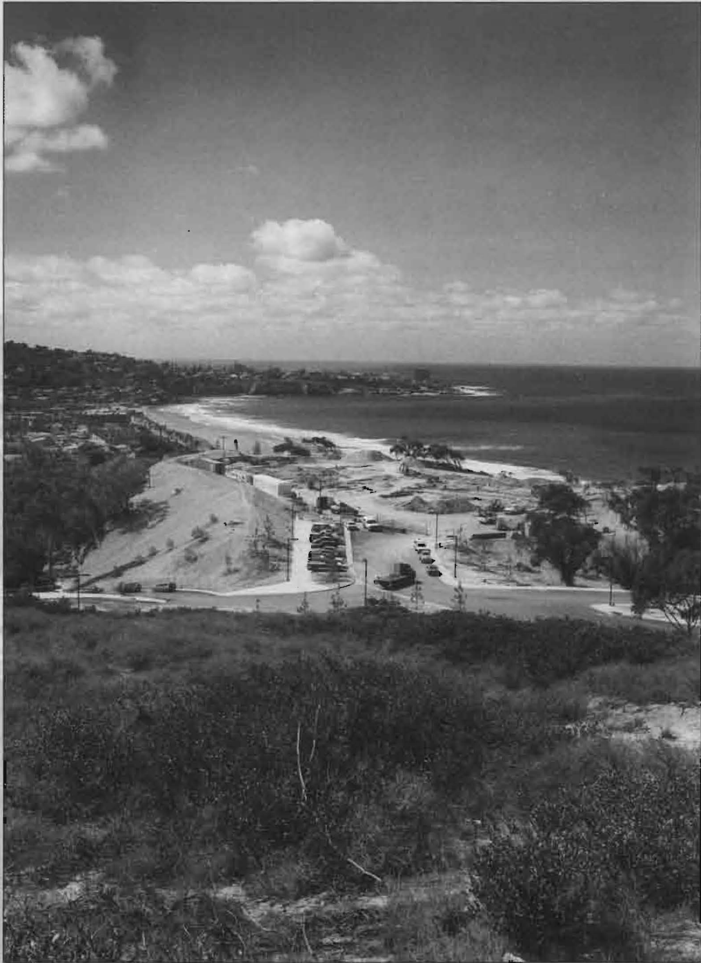
Ungraded site of the Stephen Birch Aquarium-Museum, the Scripps campus in background.
