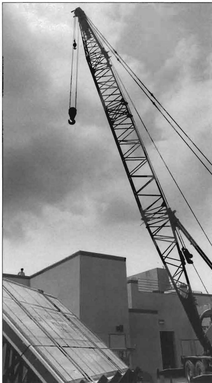
The kelp forest exhibit window, California's largest acrylic viewing window, being readied for placement by a giant crane.
