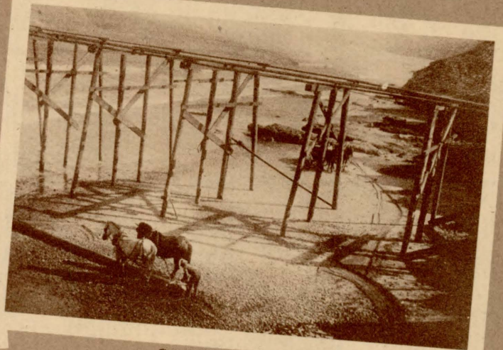
Scripps Pier under construction, 1915-1916.
