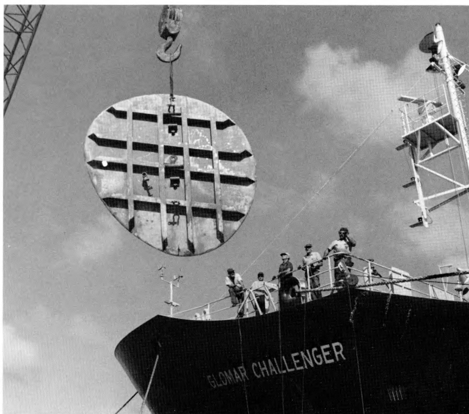
When ship personnel inspect or repair thruster system of D/V Glomar Challenger , a circular piece of equipment, called a coffer dam, is used to shut off flow of water into the ship's forward thrusters. Here, the "dam" is being lowered into place during vessel's port stop at San Juan, Puerto Rico, harbor.
