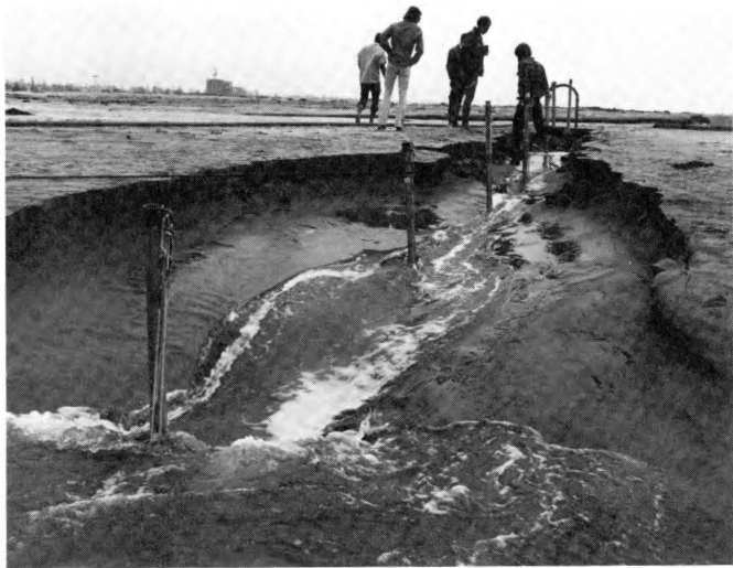
Shore Processes Study Group team conducts field test of 20-m-long fluidizing pipe at Oceanside Harbor. Vertical pipe supports protruding through sand maintain fluidizing pipe at a fixed depth while it transports sand. Trench was excavated by fluidizer in 20 minutes after saturation of sand with water. Shore Processes Study Group
