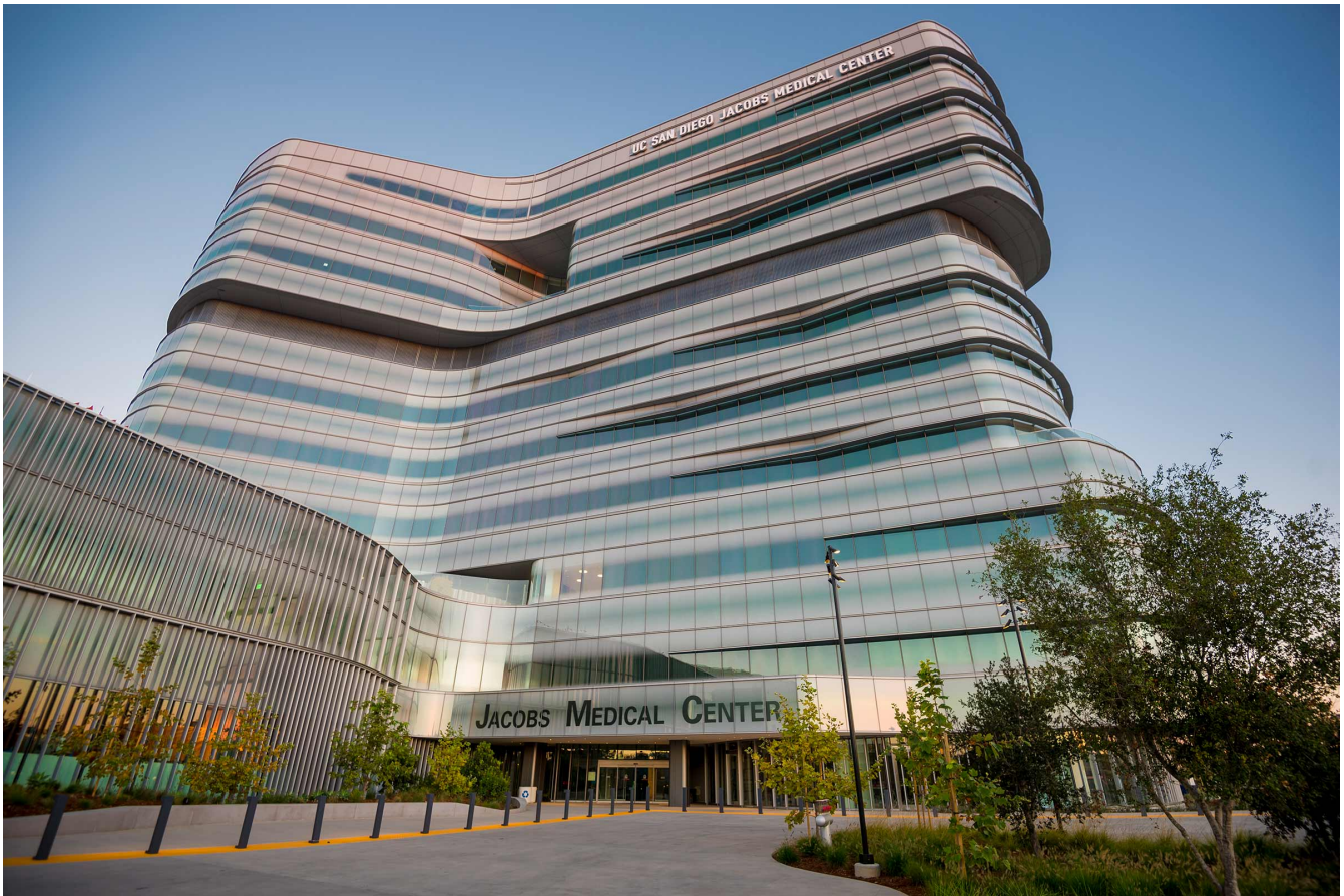
Exterior view of the 10-story Jacobs Medical Center at UC San Diego Health. Photos by Erik Jepsen/UC San Diego Publications
