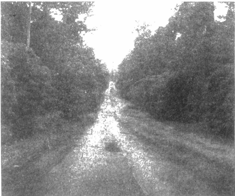
National Programming System requires the reporting to NMA of projects in the provinces like this road from Vanimo Township to the PNG/Indonesia Border.
