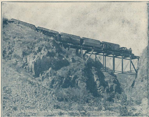
High Bridge, Sweetwater River
