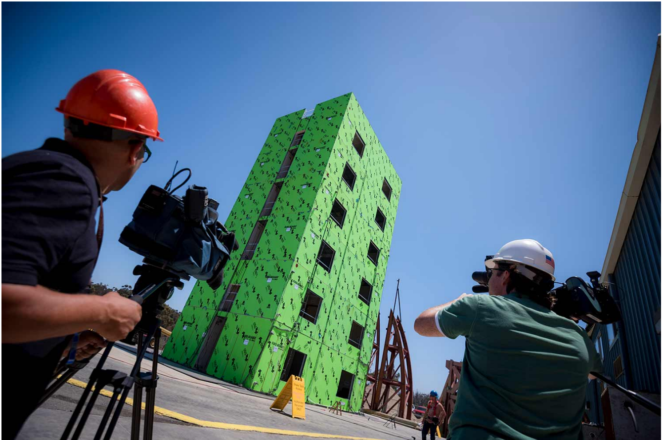
Researchers tested a six-story steel frame building in 2016. Photo by Erik Jepsen/UC San Diego Publications
