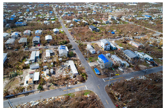
Loss of wetlands caused about $430 million more in damages from Hurricane Irma.
