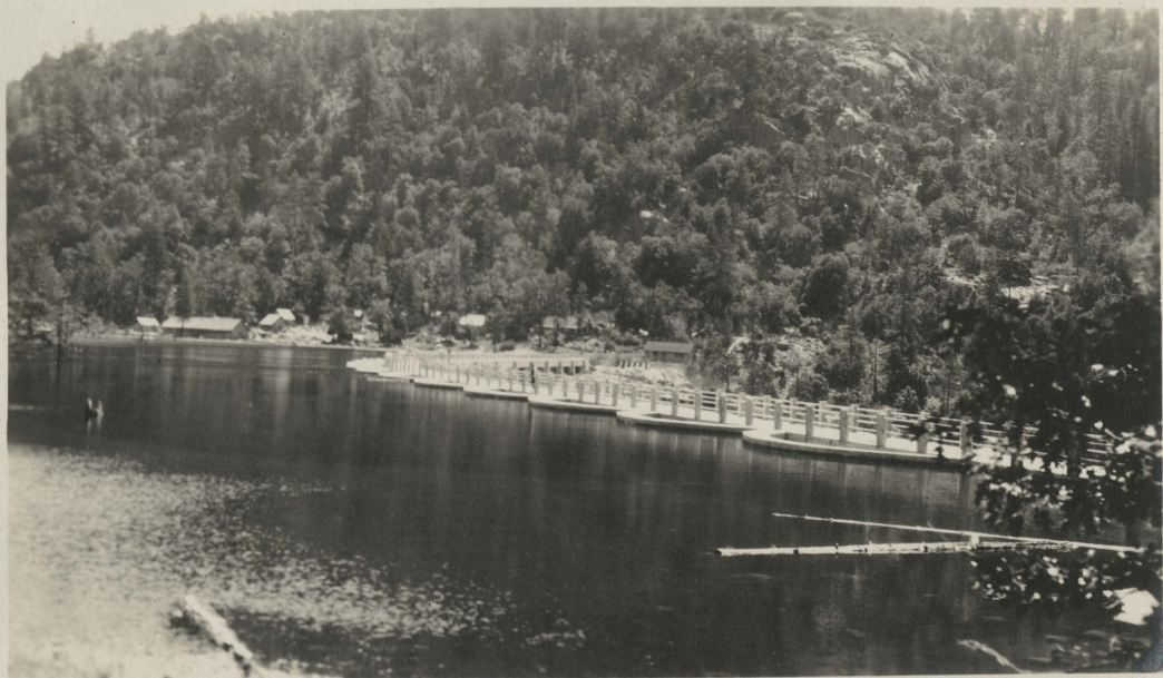
Lake Eleanor Multiple Arch Dam
