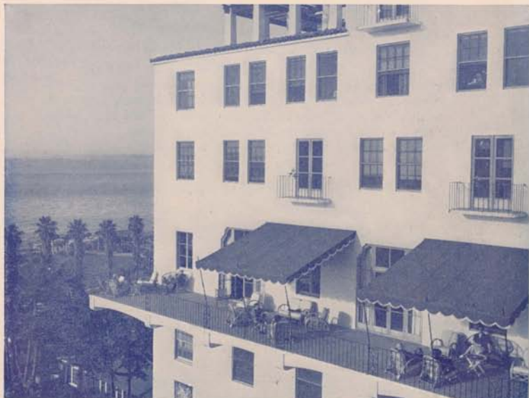
La Valencia, Showing Sun Balcony and Terraced Garden
