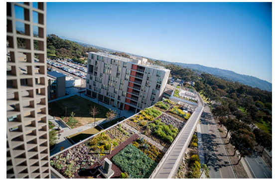
Green Building Tours reveal how the campus creatively employs sustainable design techniques, like the Keeling Apartments in Revelle College. Photo by Erik Jepsen, UC San Diego Publications.
