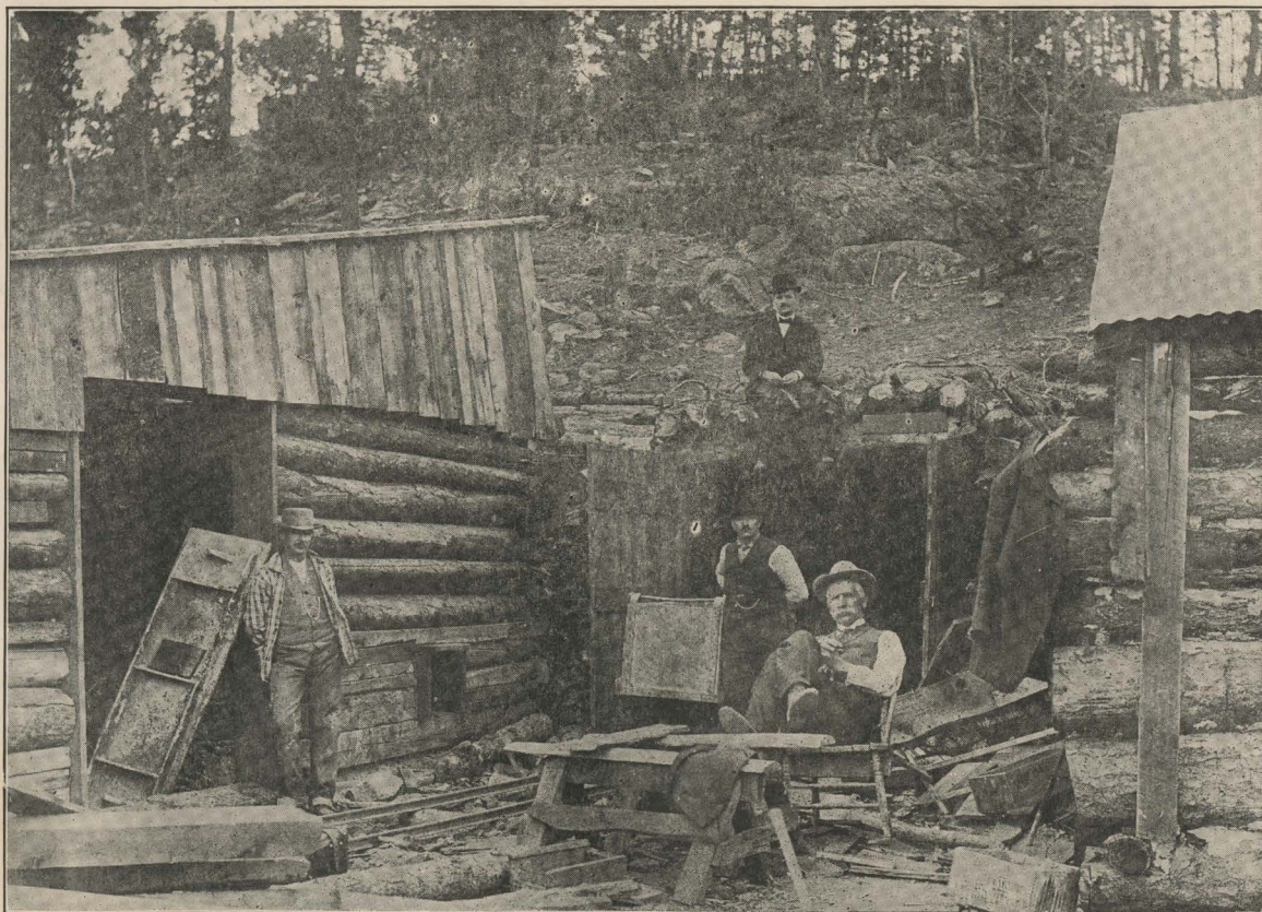
SHOWING TOOL HOUSES, ETC., AT MOUTH OF OUR TUNNEL
