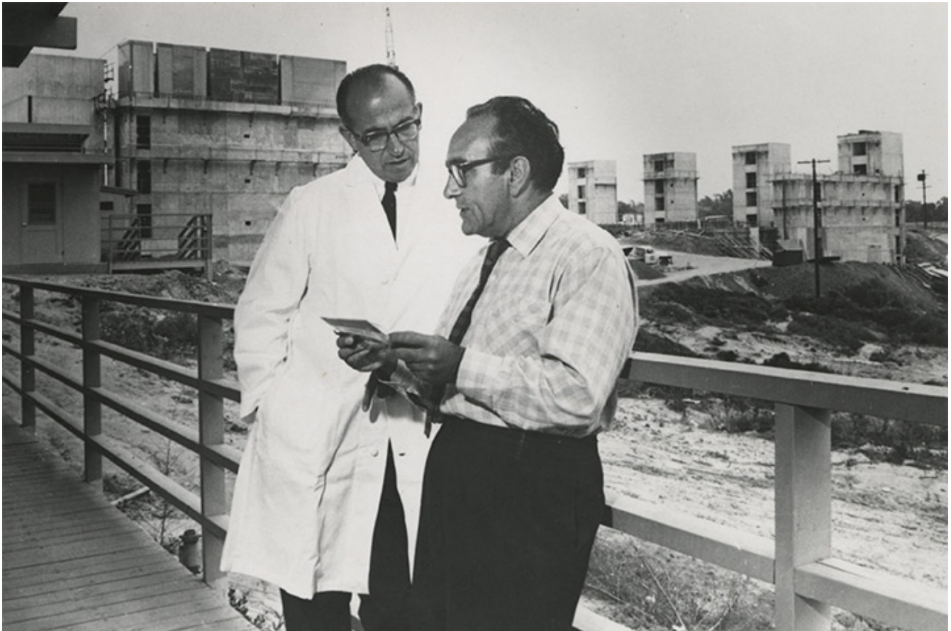
Jonas Salk (left) with Jacob Bronowski in front of the Salk Institute, during construction.
