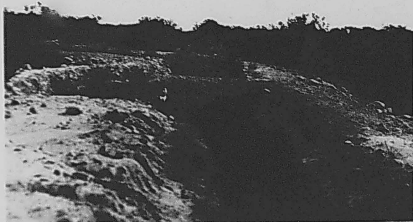
Photograph showing depth of trenches.
