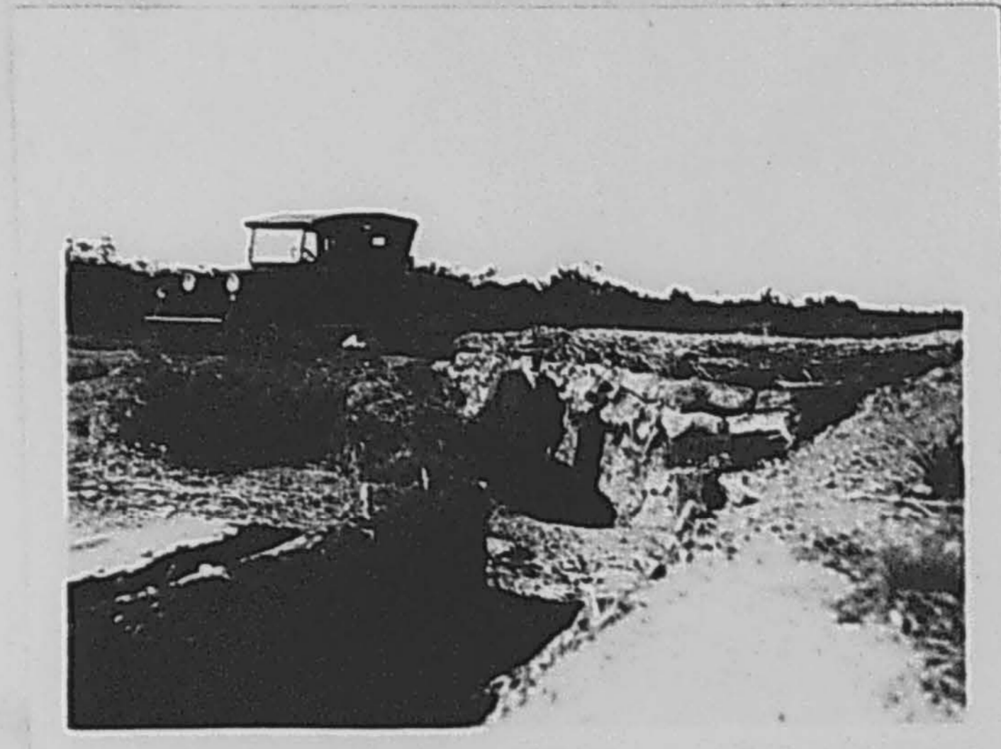
Photograph showing 400 feet of trenches.
