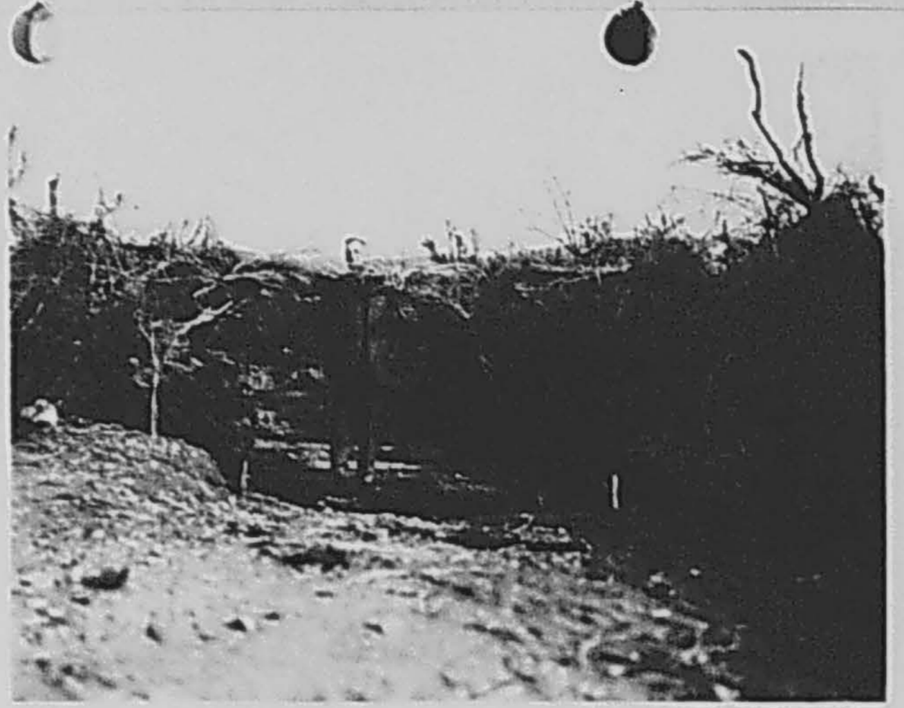
Photograph showing observation excavations 30 ft. wide and 6 ft. deep - camouflaged.
