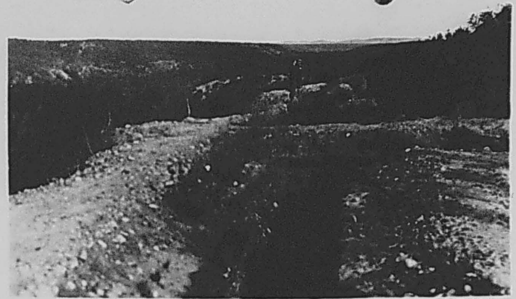
Photograph showing inter-communicating trenches.
