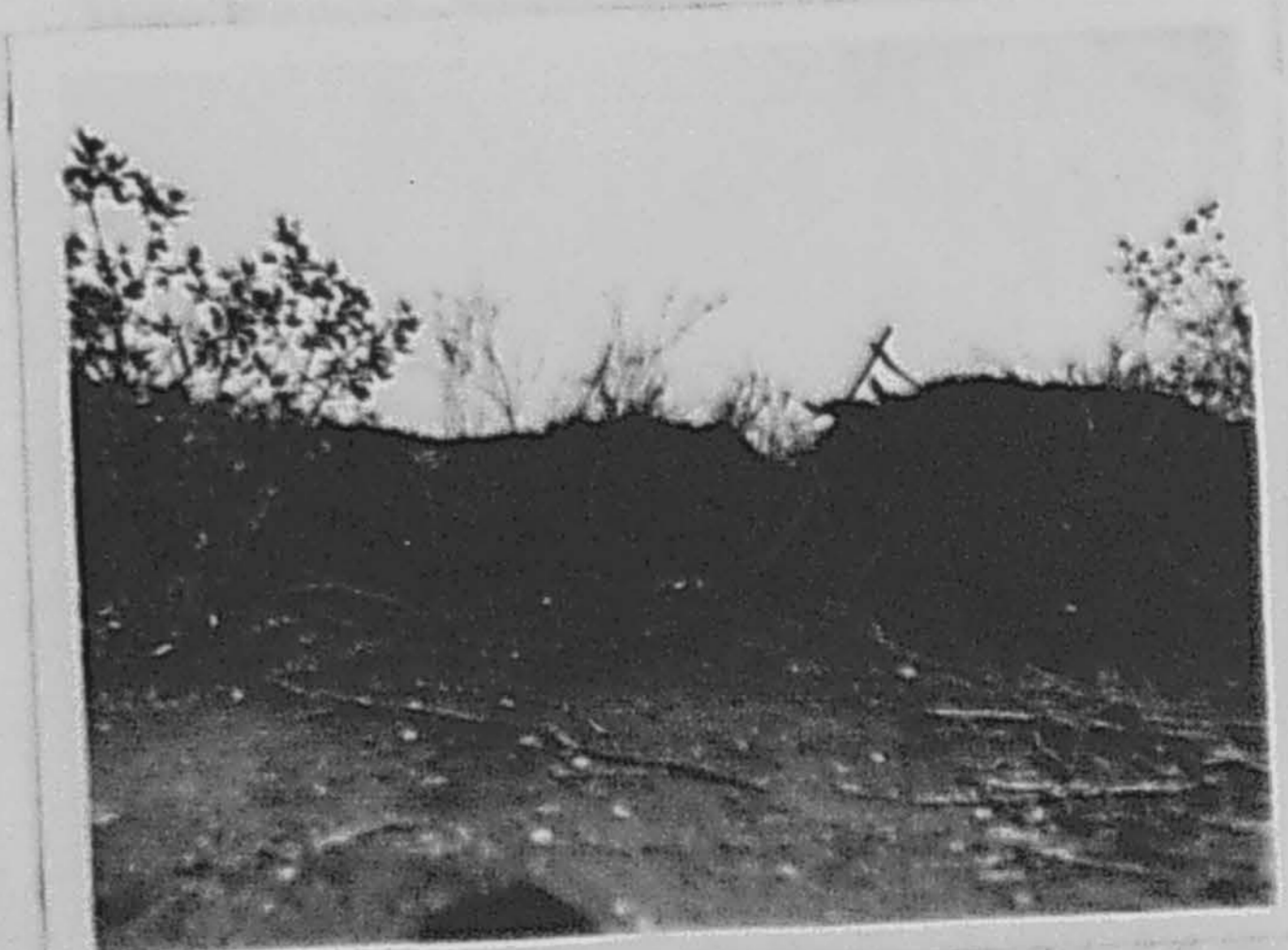
Photograph showing observation excavations.
