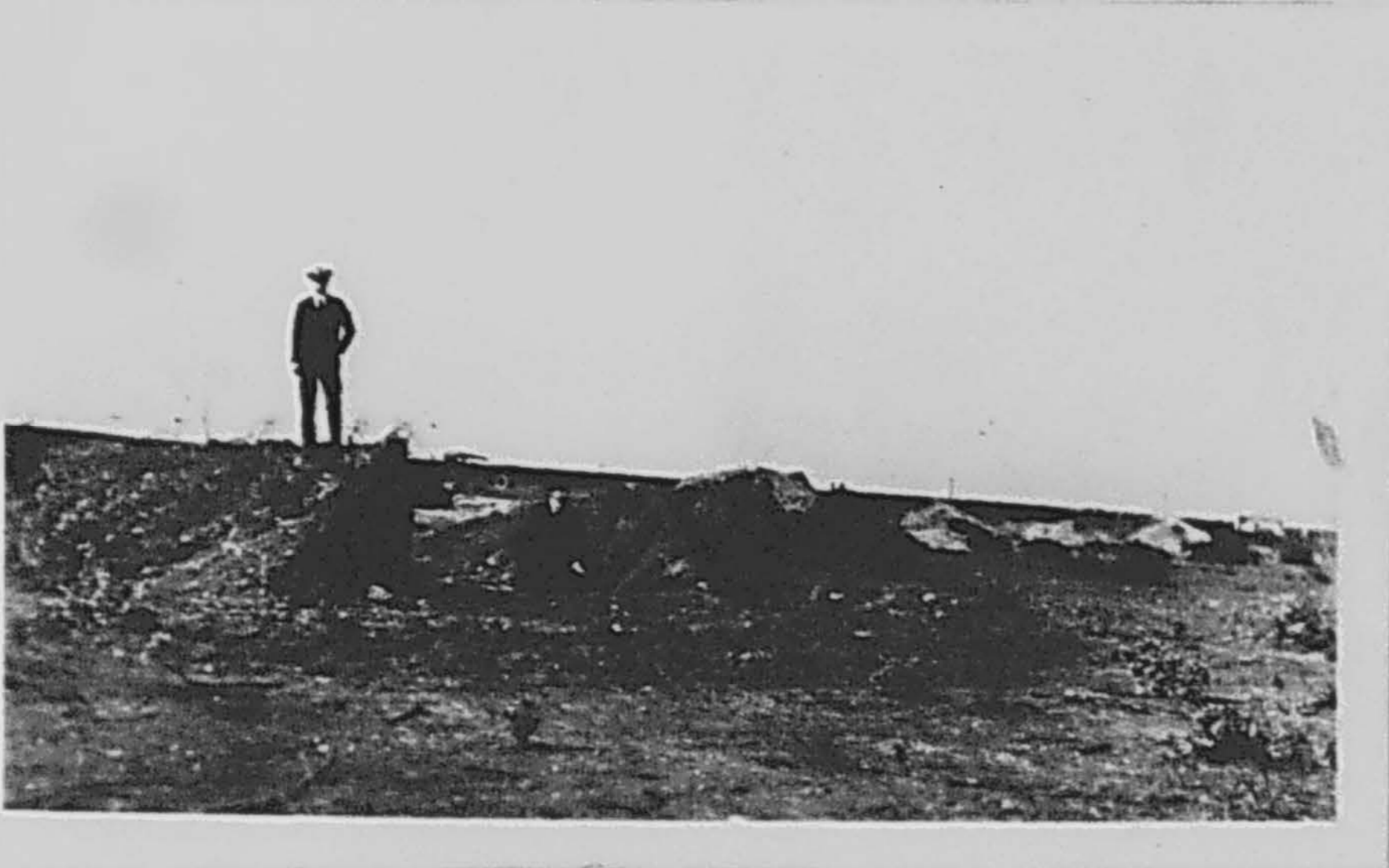
Photograph showing 800 ft. of excavations and embankments for guns.
