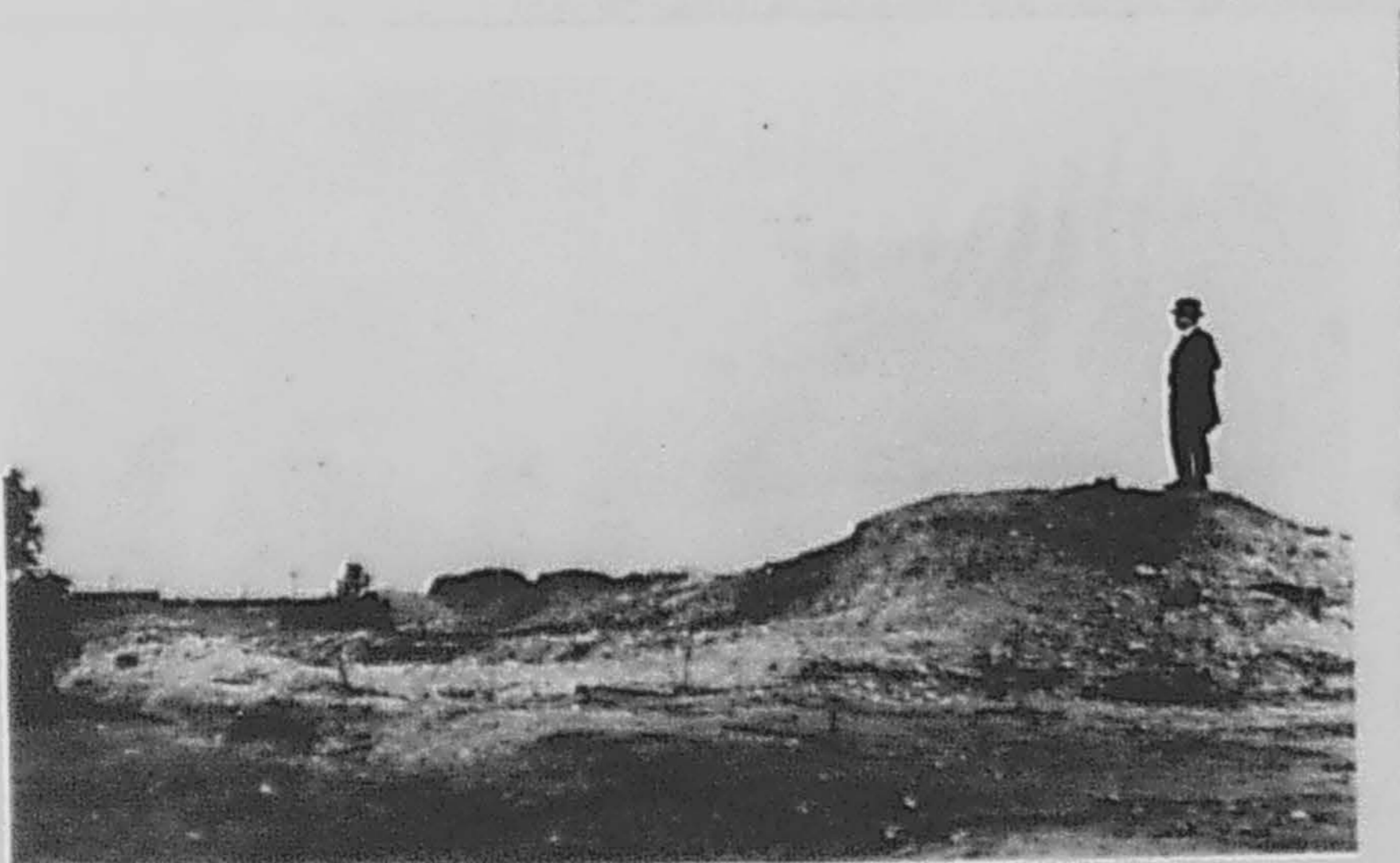
Photograph showing 8 ft. embankment.
