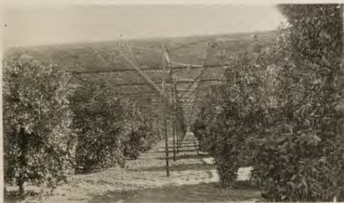
Covering shown from beneath.
