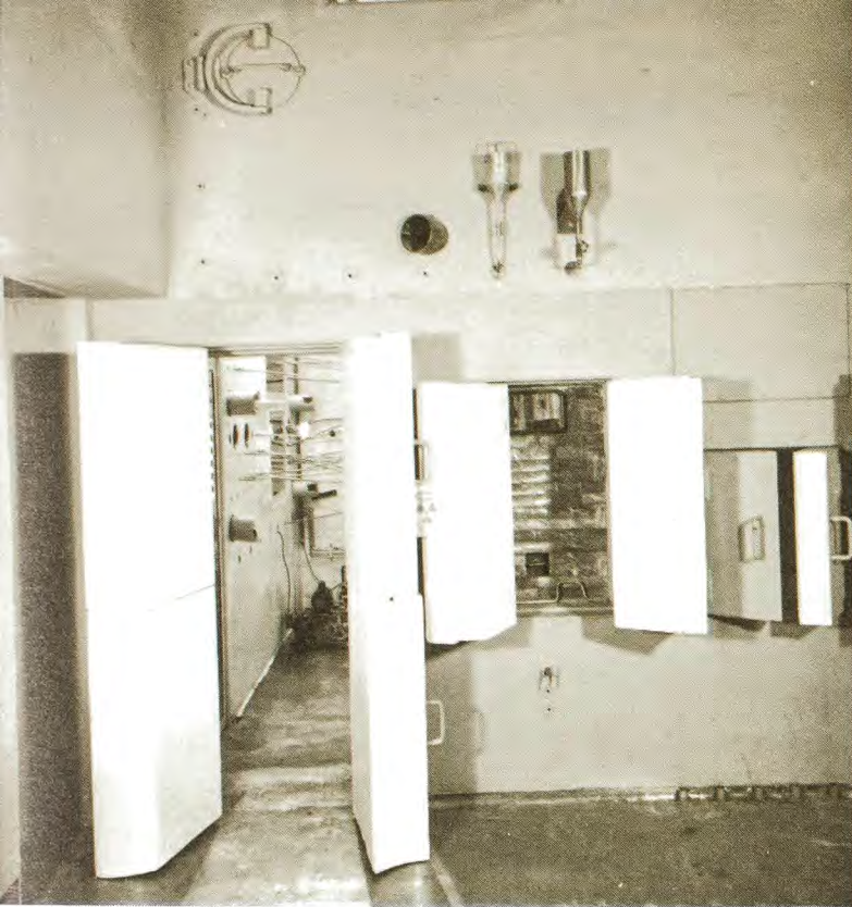
A "hot cell" for kilocurie fission product separation. The view is into the side of the cell, the heavy, white-painted lead doors of which have been swung open. Through the larger doors one sees the inside of the control face of the cell, and the slender horizontal rods serve for the remote turning of valves and for other manipulations on the apparatus, which is hidden from view to the right of the large door.
