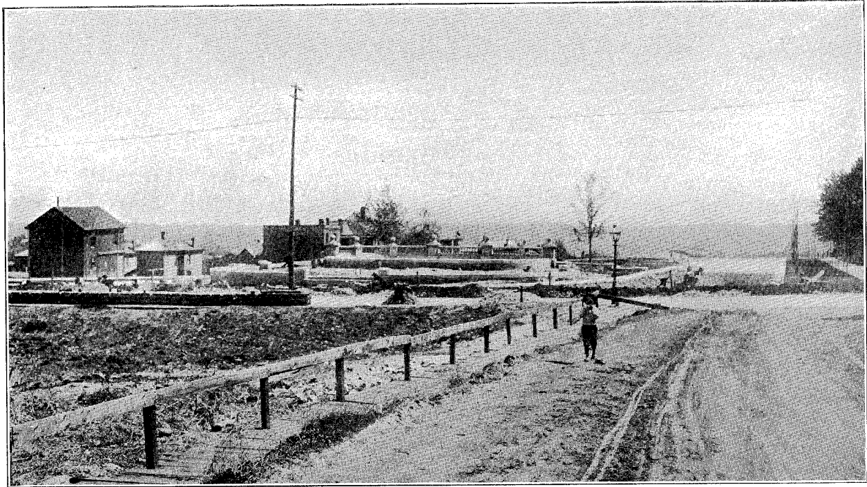
THE PASEO, KANSAS CITY, MISSOURI. FOUNTAIN UNDER CONSTRUCTION.
