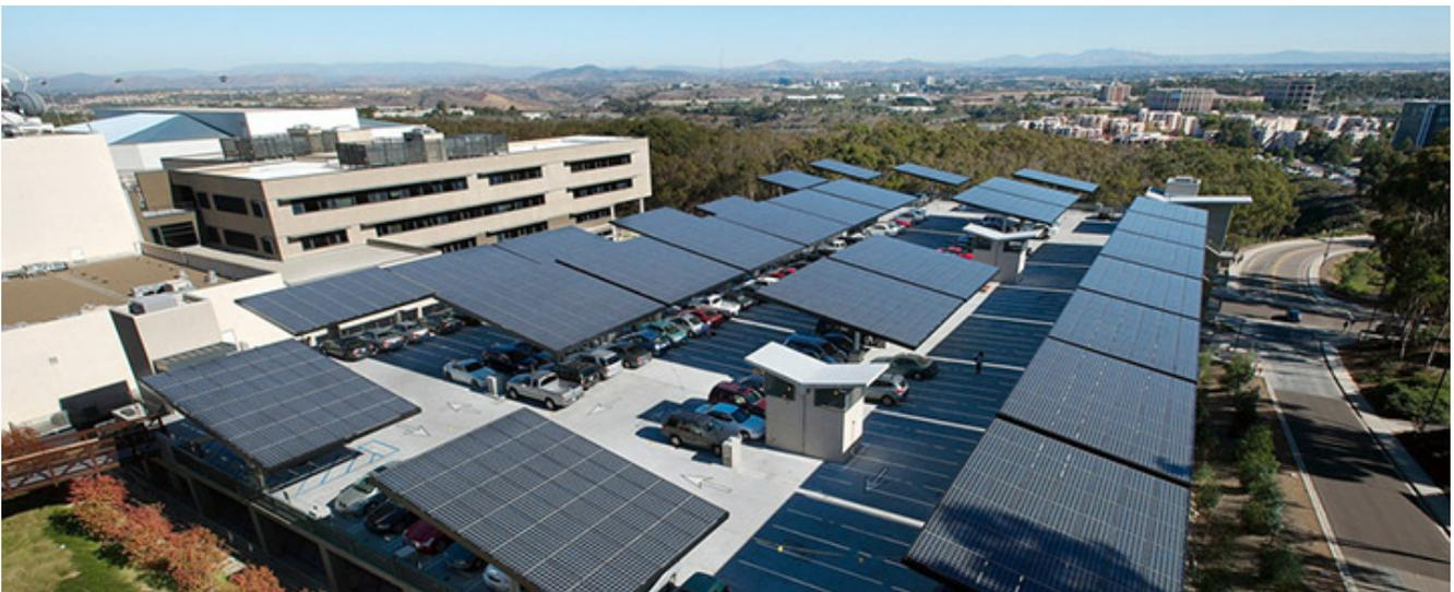
*Solar panels like the ones perched atop the Hopkins Parking Structure are part of the UC San Diego microgrid, which generates 92 percent of the electricity used on campus.*
