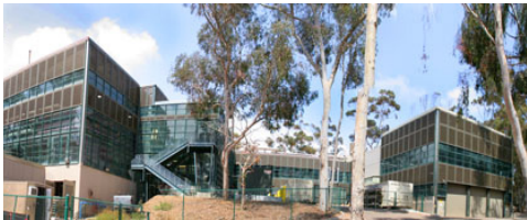
UC San Diego's highly efficient natural gas-fired cogeneration plant will now have emergency restart capabilities.
