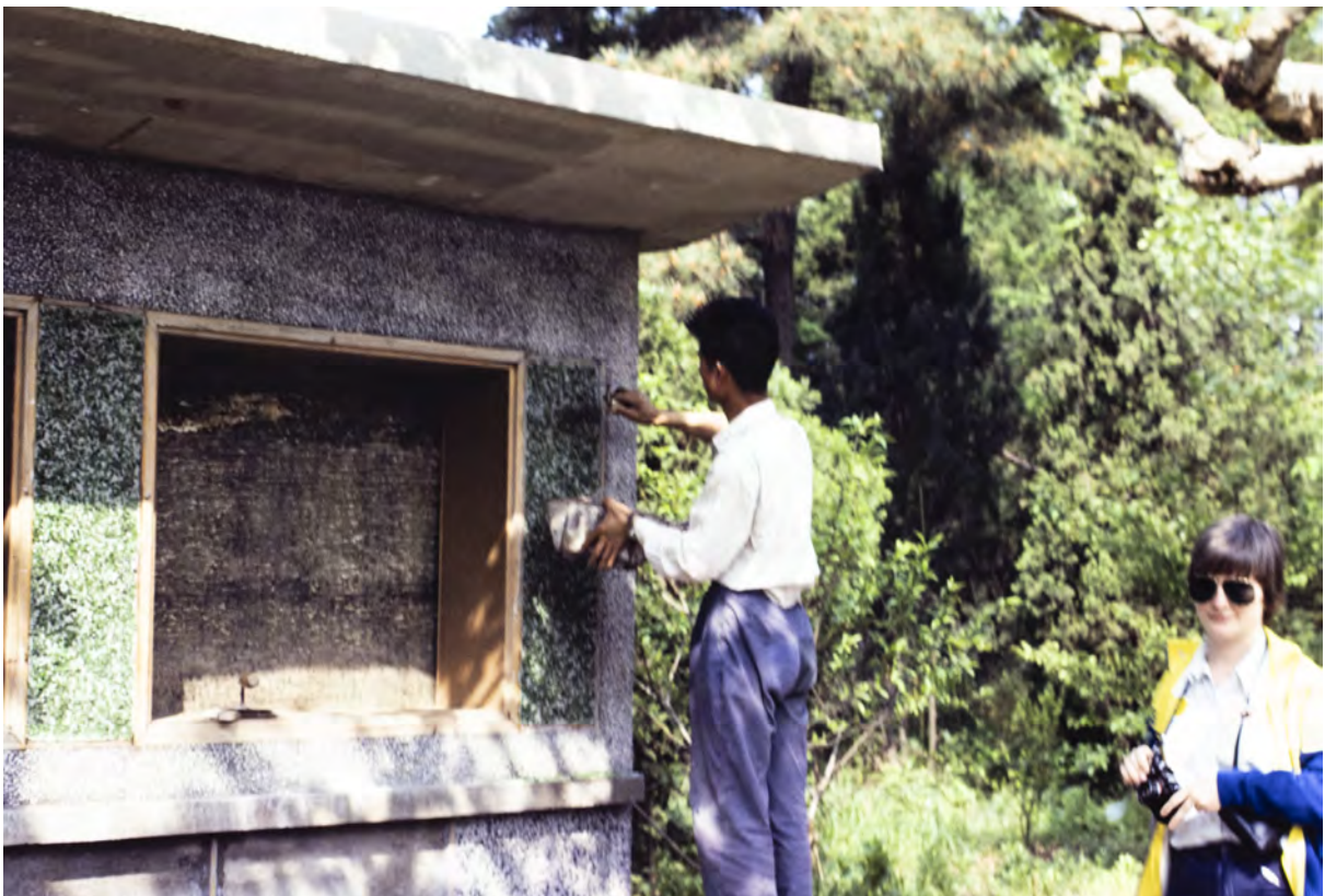
Repair at sanatorium
