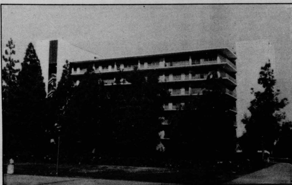
More than $100,000 have been requested for improvements for the ventilation systems of Urey Hall.
