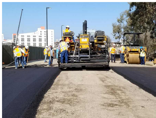
Crews install the asphalt which replaces tar-based bitumen with recycled plastic.
