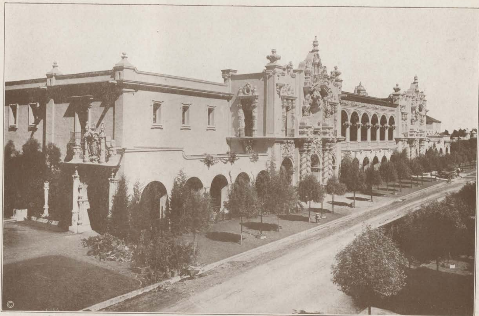
Varied Industries Building, from across El Prado—San Diego Exposition. Photo Supplied by Underwood & Underwood, N. Y.
