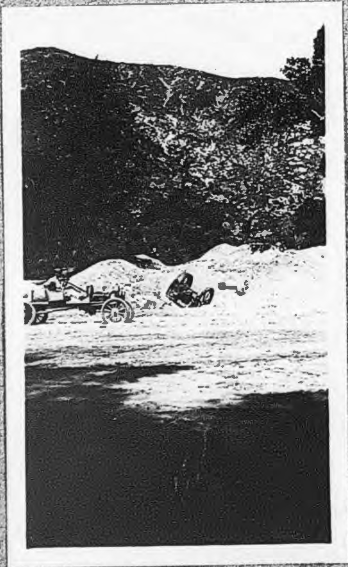
Damage to Sand Creek Pumping Plant.
