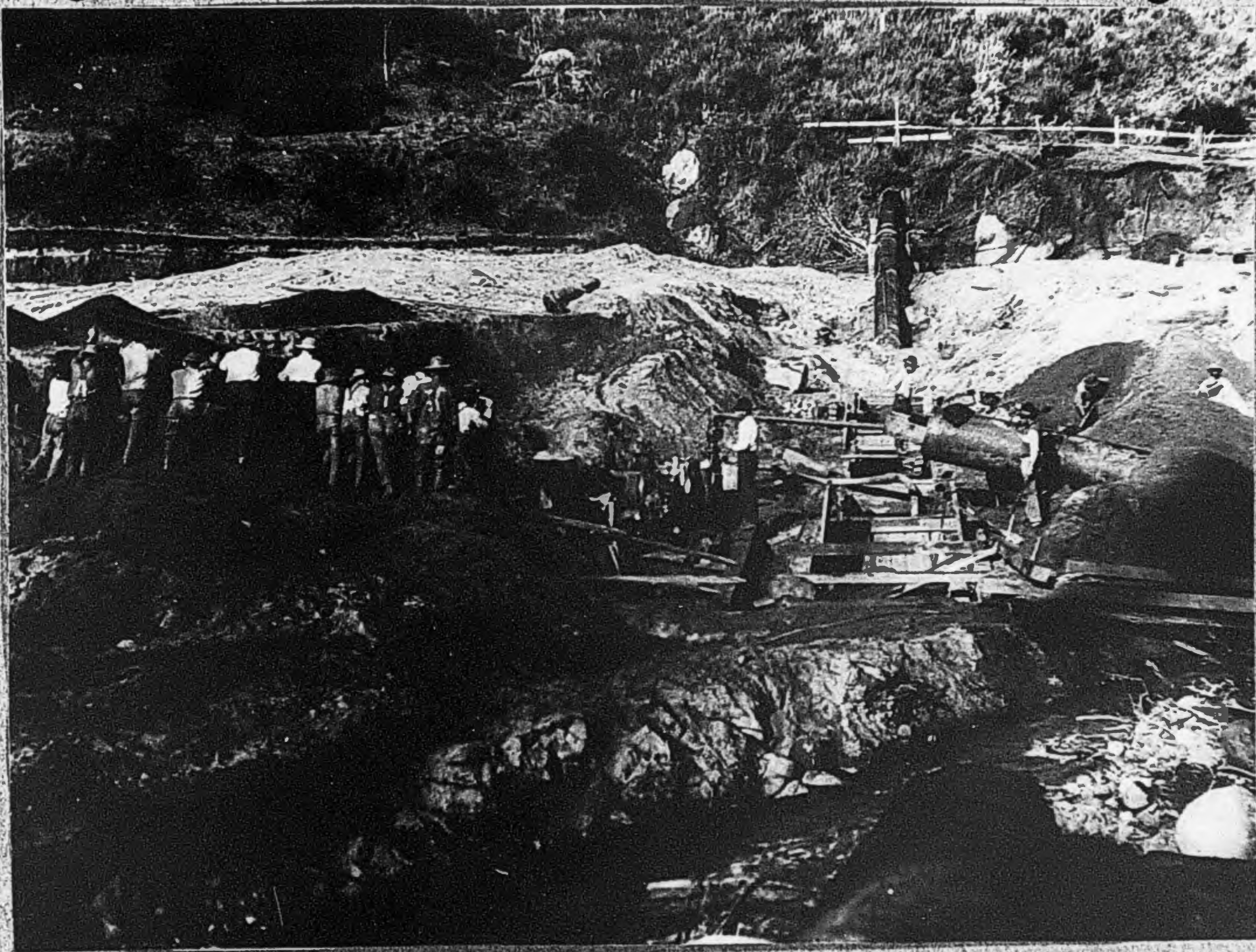
Repairing Chocolate Siphon. Note Sheet Piling, Pump and Diversion of Creek.
