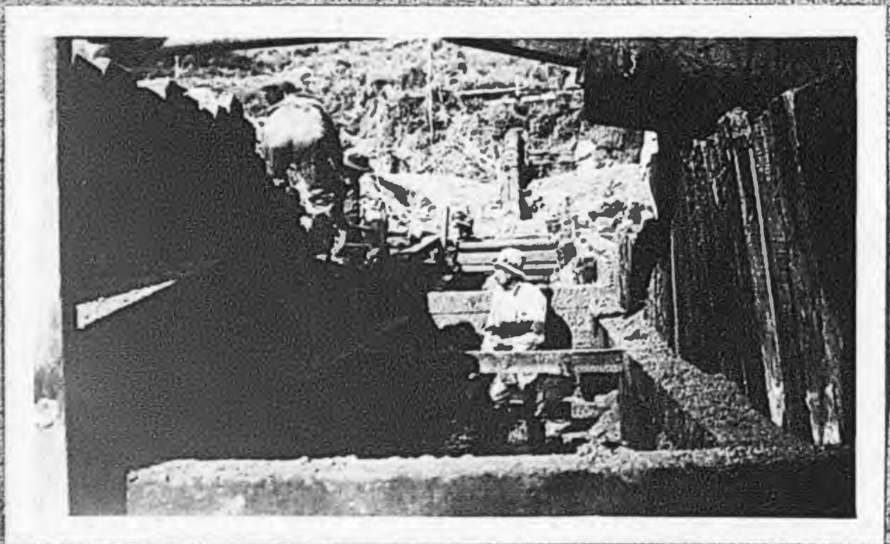
Repairing Chocolate Siphon.
