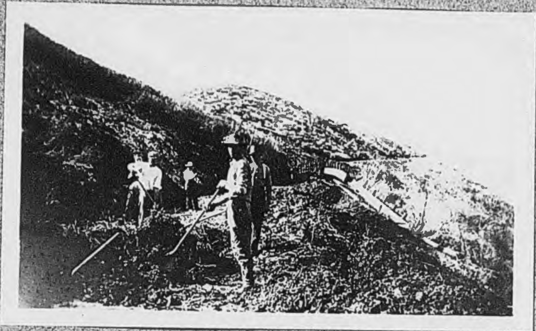
Repairing Main Flume
