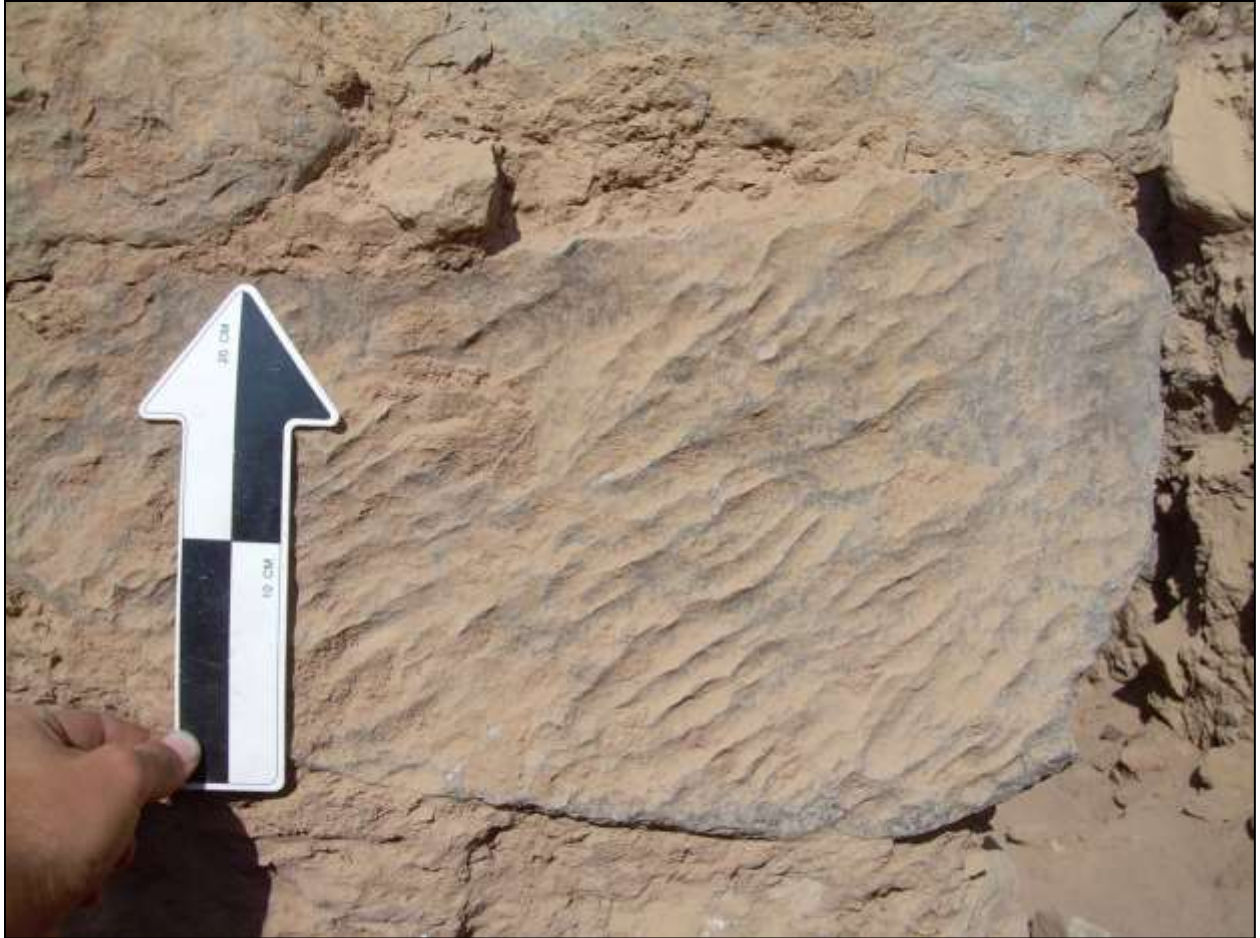
Figure : Possible tool marks running diagonally across one face of a dolomite building stone in the northeast corner of wall locus R09L086.
