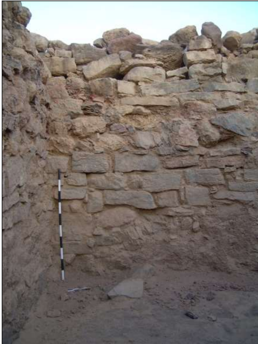
Figure : The northwest corner of Room 5, displaying construction technique of wall locus R09022.
