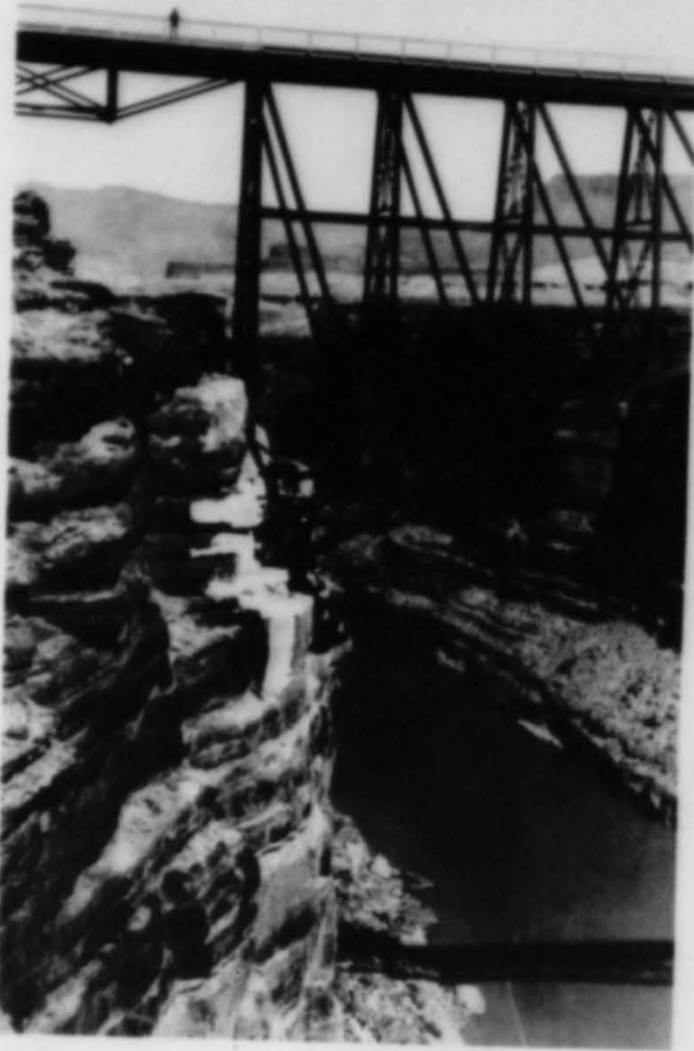
Bridge 456 feet above water 568 feet long
