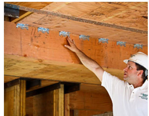
John van de Lindt, a professor at Colorado State University, the lead investigator on the tests, shows some of the seismic retrofits the building is equipped with.
