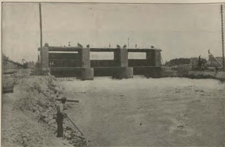
View of Headgates Laguna Dam Looking North
