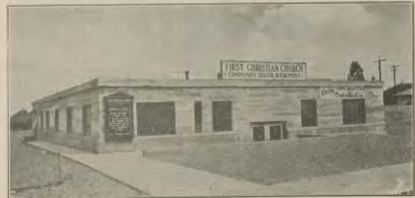
First Christian Church of Yuma, Basement Only Completed
