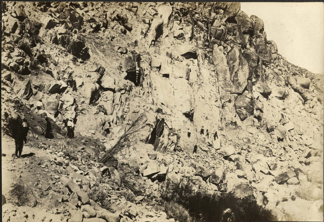
The road in the making.
