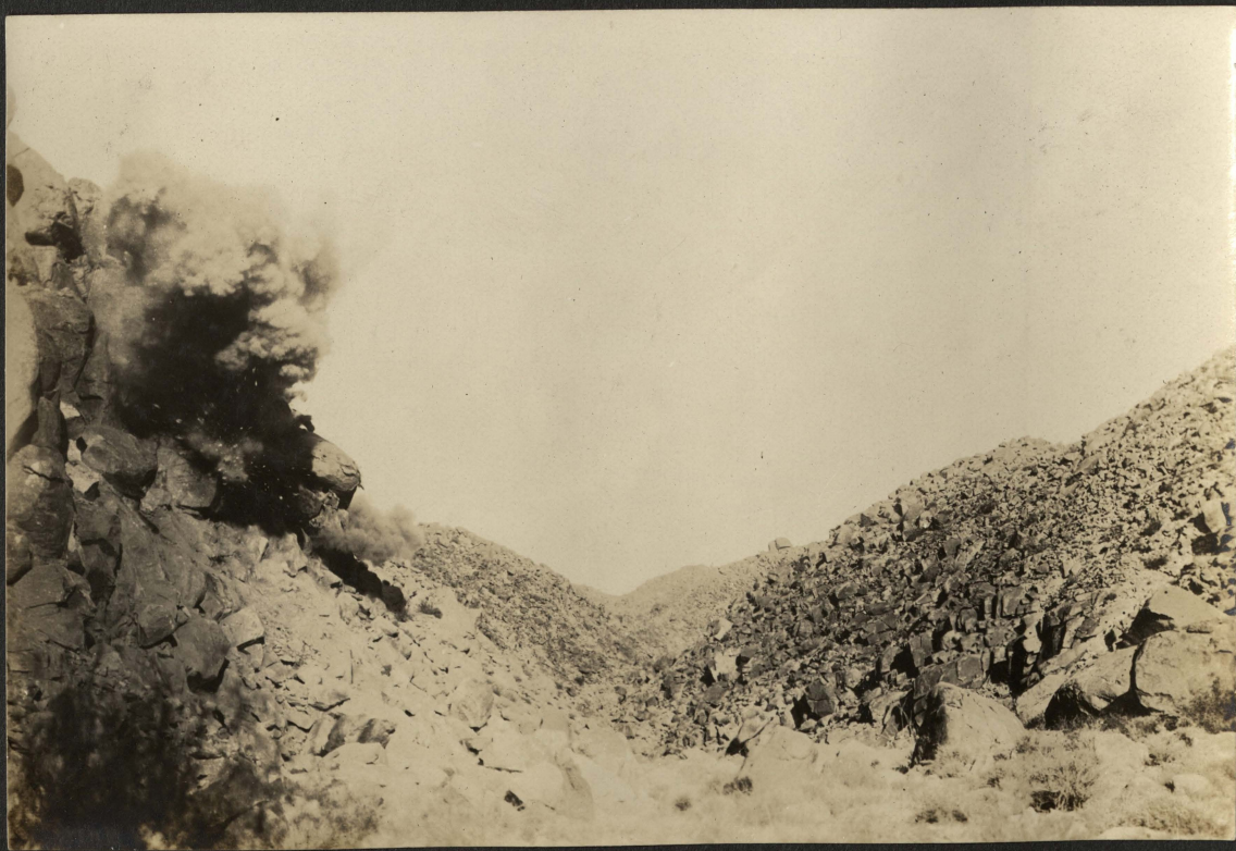
Blasting a road to the desert.
