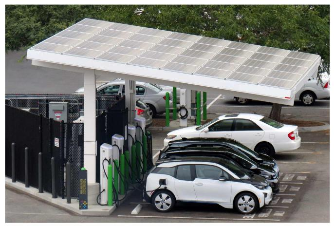
The UC San Diego/EVgo project combines the fastest electric vehicle charging technology, second-life battery energy storage and integration of solar energy to mitigate impact on the UC San Diego microgrid.
