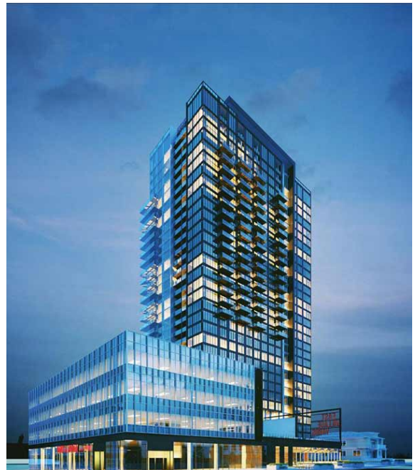
The 66,000 square foot center, part of a larger project at the location, will offer educational and cultural programs.
