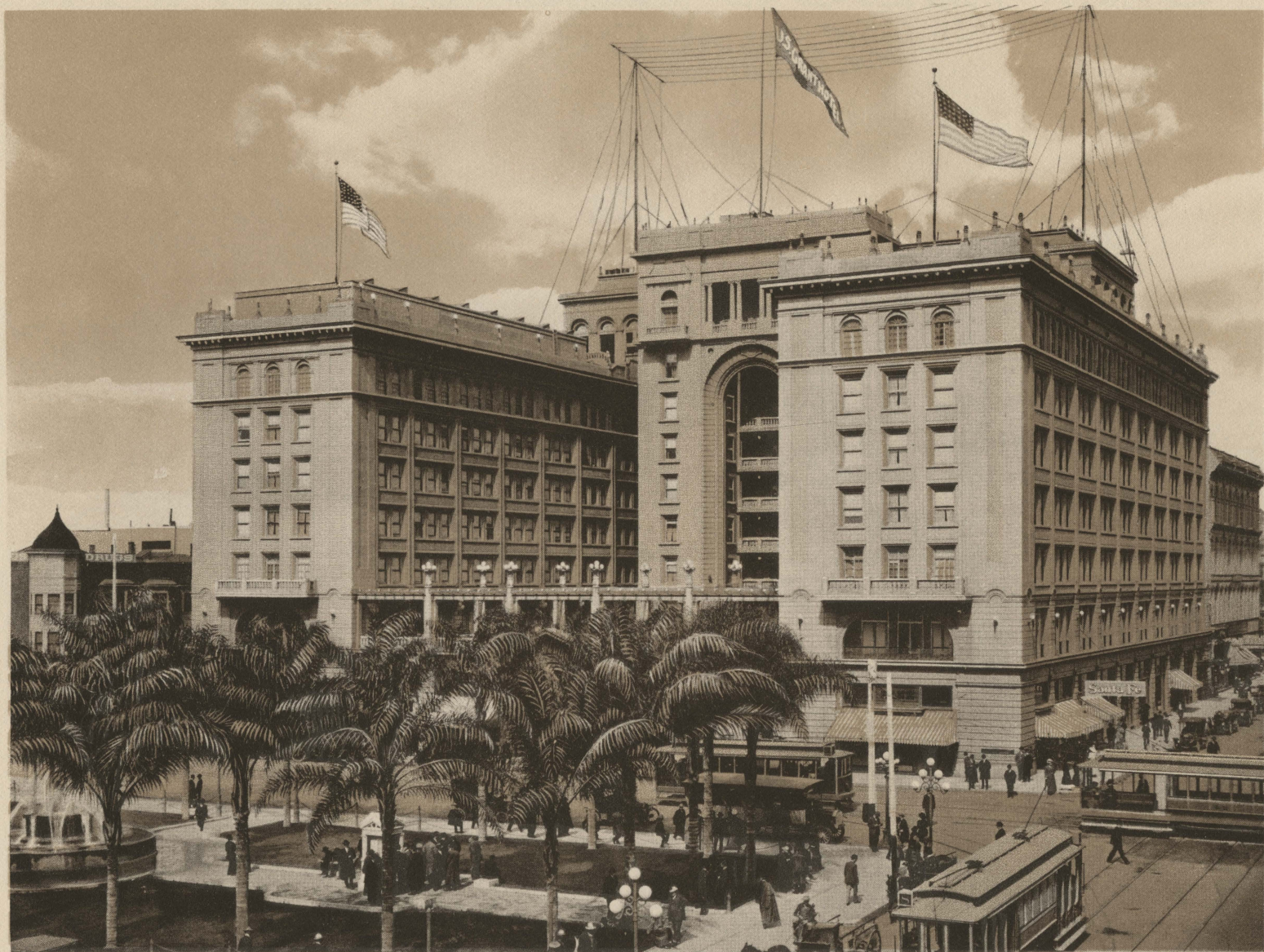
U. S. Grant Hotel, facing Plaza Park. Constructed at a cost of $2,000,000. Erected by U. S. Grant, Jr. as a memento to his father General U. S. Grant.
