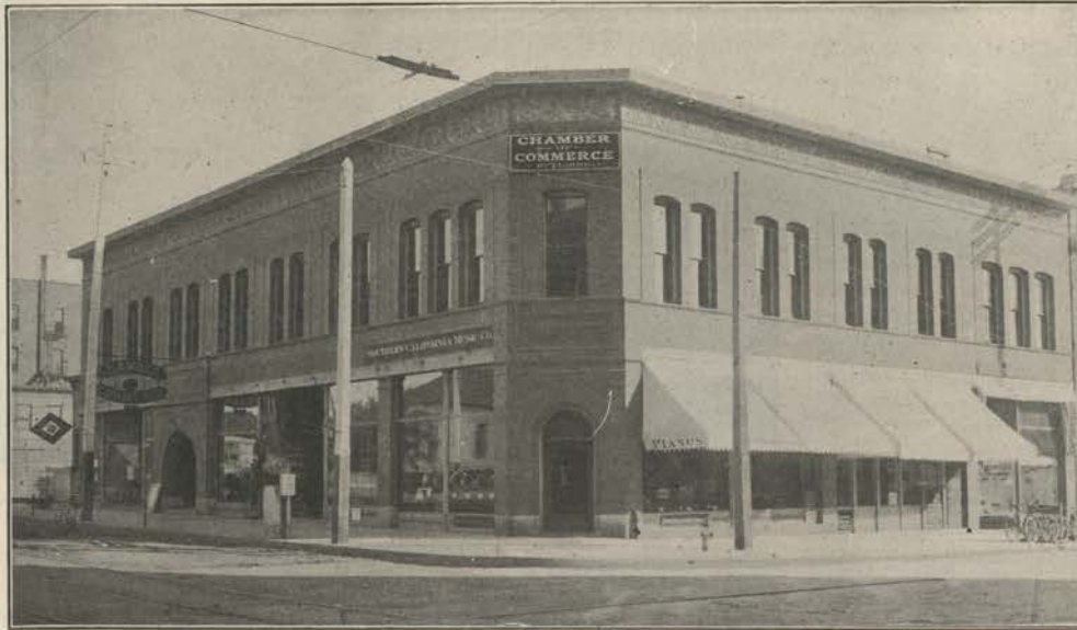
CHAMBER OF COMMERCE BUILDING
