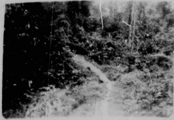
PART OF ROAD BEING CLEARED
