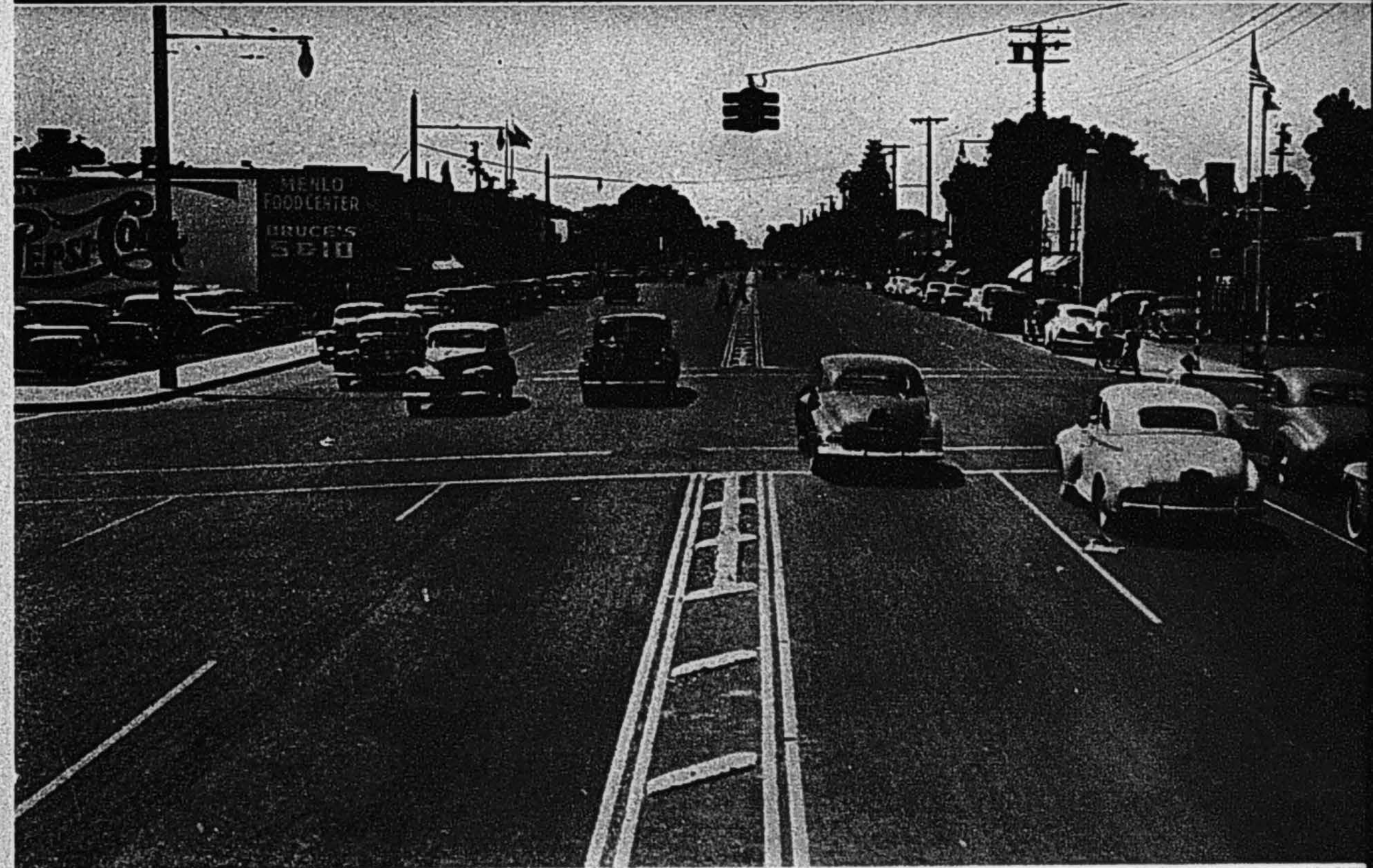
Top, improved section of U. S. 101 showing channelized division strip approaching Atherton. Below, widened avenue through Menlo Park
