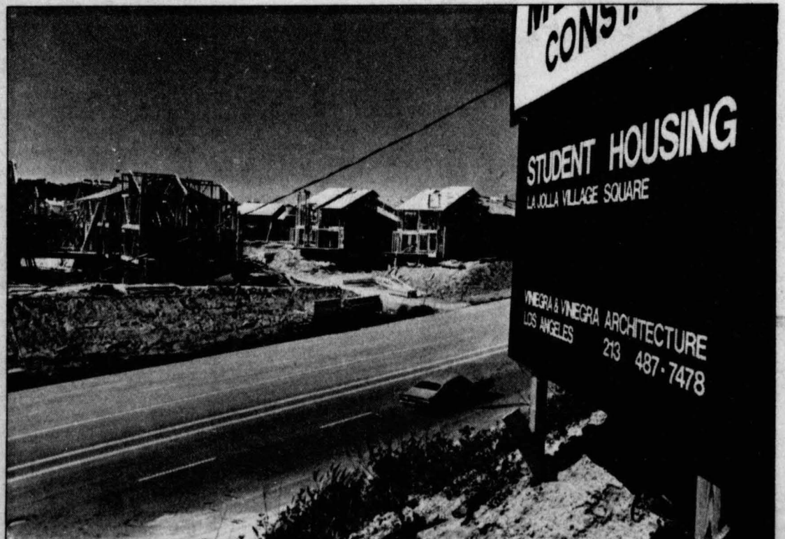
Condominiums under construction on Via La Jolla Dr., south of UCSD.
