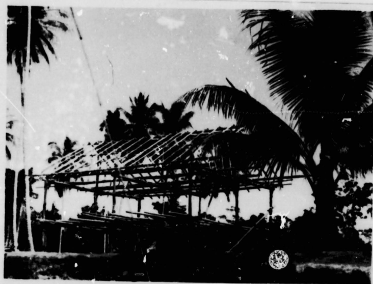
HOUSE UNDER CONSTRUCTION SIS VILLAGE
