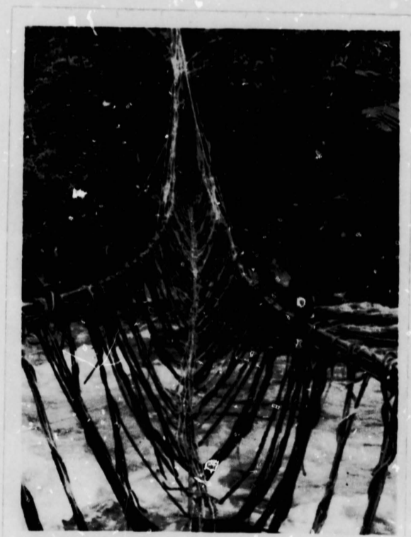
67. Suspension bridge over GIUMU at Sedema.
