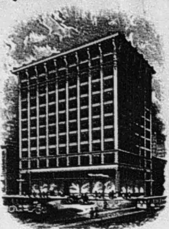
W. I. HOLLINGSWORTH BLDG. COR. 6TH & HILL ST.
