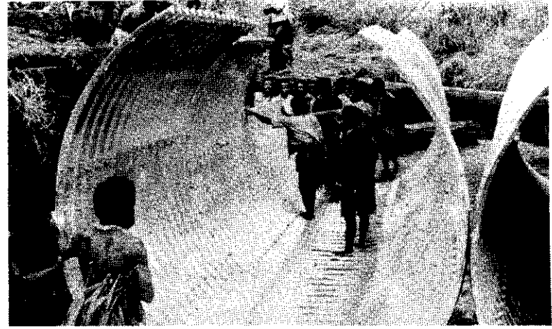
(4) Graham Campbell, em i wanpela ensinia, i wok hia wantaim ol pipel bilong Saten Hailans i wokim wanpela bikpela mambu bilong wara i brukim rot i stap namel long Ialibu na Tambul. Nau wara i stap aninit long rot na ol pmv i ken ran gut.
