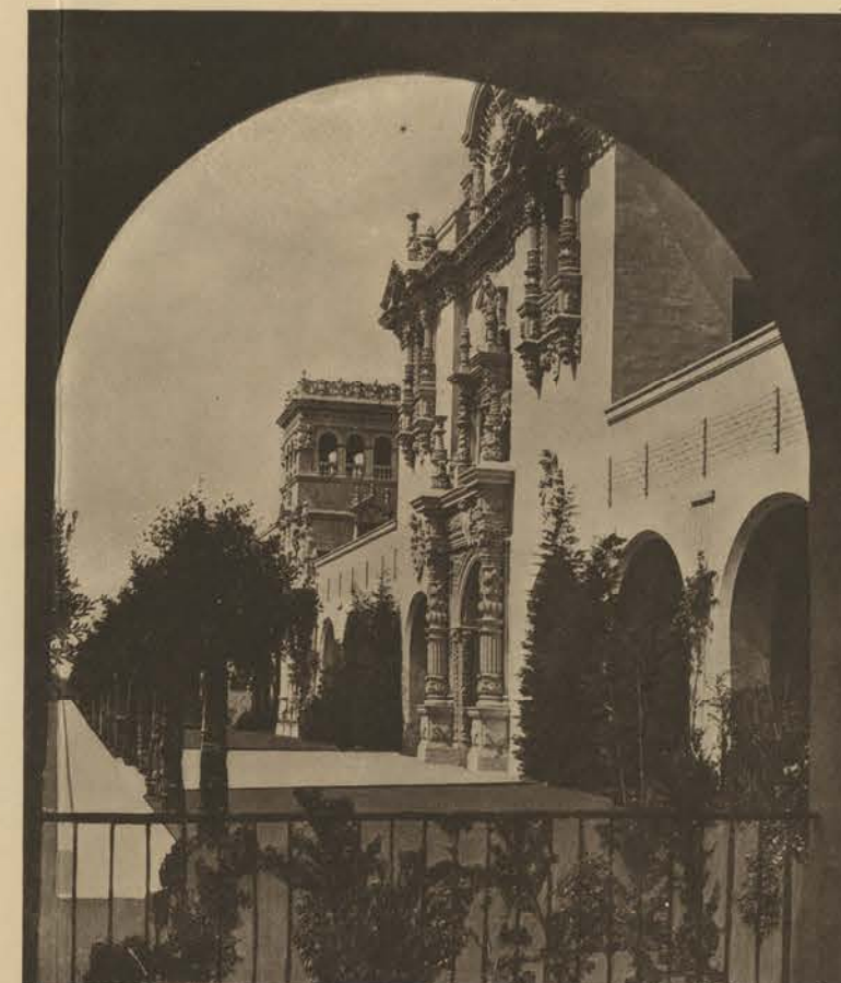
Front Entrance Foreign Arts Building.
