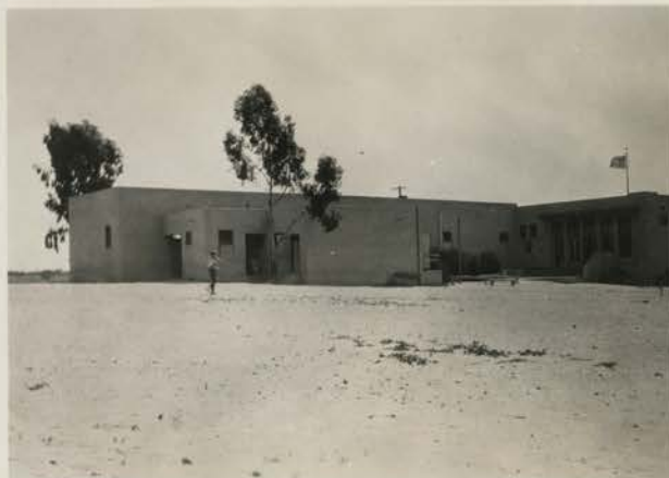
Main Building - Rear Elevation
