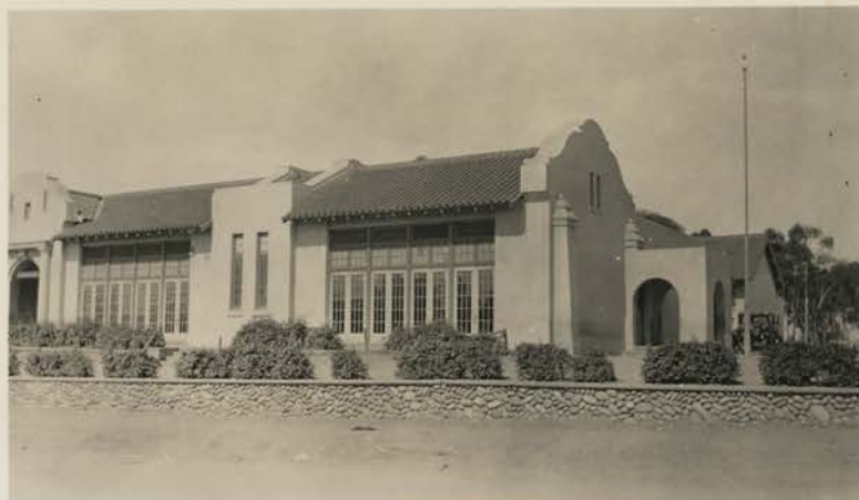
Main Building - Front Elevation
