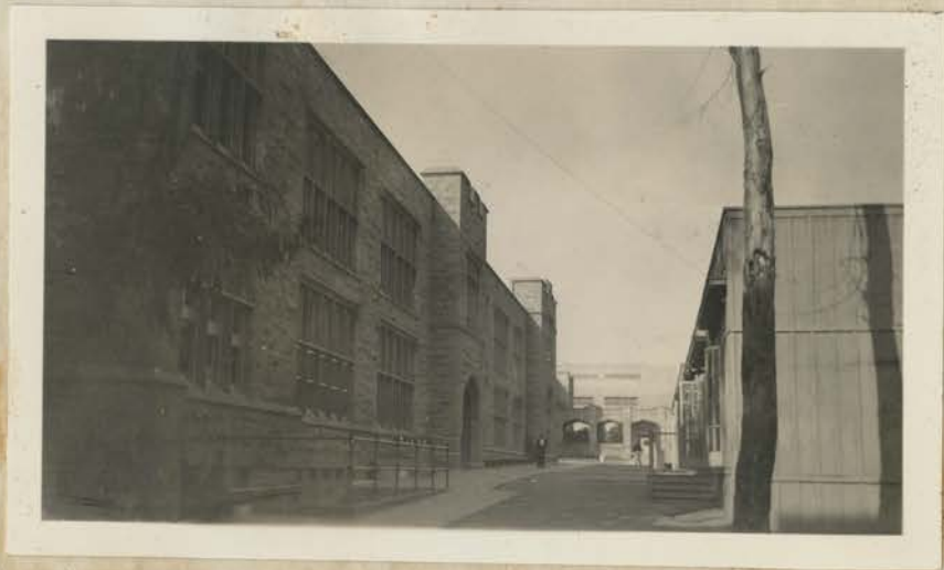
Administration Building - Rear Elevation (Temporary Buildings at Right)
