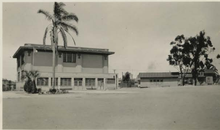
Main Building - Rear View Showing one Story Addition Bungalow - Shower at Right
