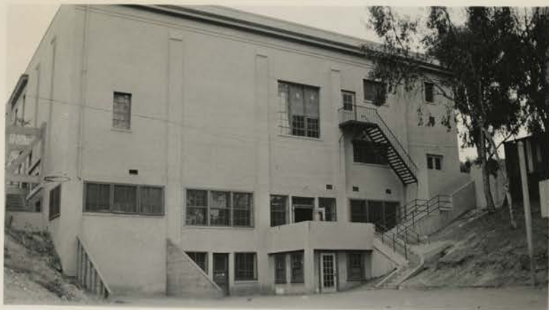
Auditorium Building - Rear Elevation
