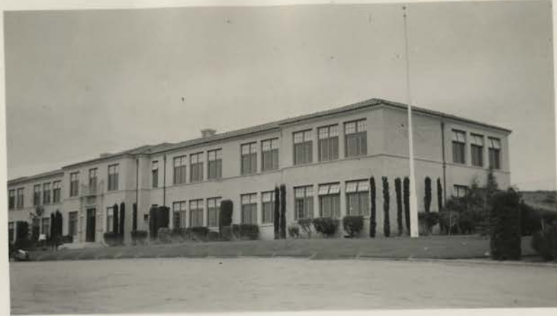
Main Building - Front Elevation
