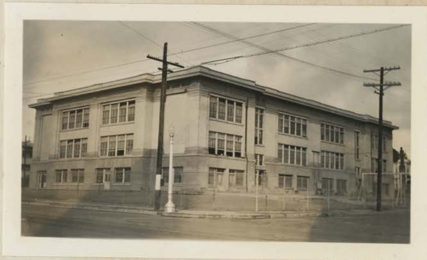
South and East Elevations
