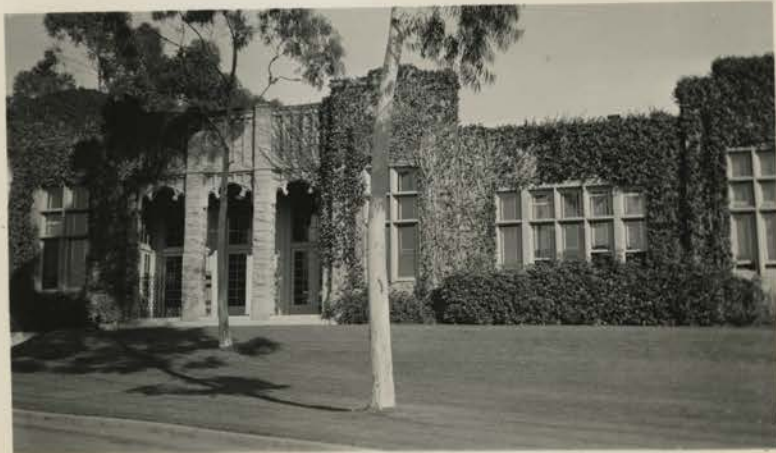
Home Economics Building - Rear Portion of West Elevation
