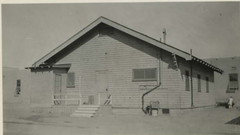
Cafeteria Building - Rear Elevation
