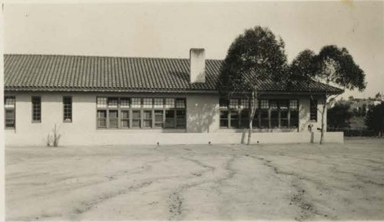
South Elevation of East Wing
