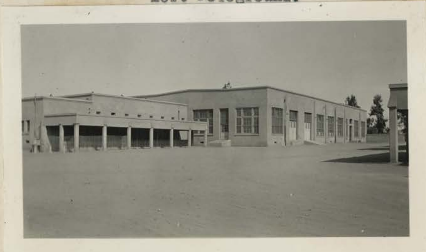
Memorial Arts Building. Side Elevation Boys' Locker and Shower Rooms at Left - Shops at Right.
