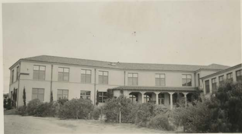
Main Building - West Elevation Showing the Shop Wing
