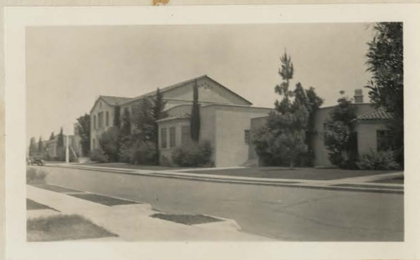
Main Building - Front and End Elevations Kindergarten Wing at Right.
