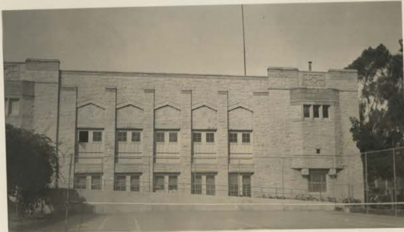
Technical Building - South Elevation
