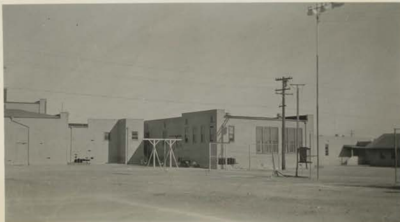
Main Building - Rear Elevation of Original Section
