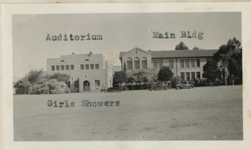
Main Building - Rear view Showing the Classroom Section at Right, Auditorium Wing at Left Back- ground, and Girls' Shower and Locker Wing at left Foreground.
