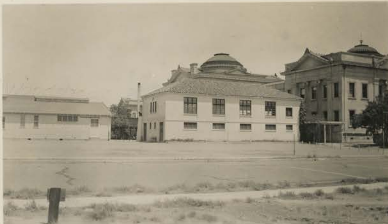
Main Building - Rear Elevation at Right Physical Training Building in Center Shop Building at Left
