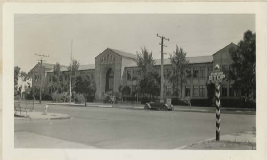
Main Building - Front Elevation
