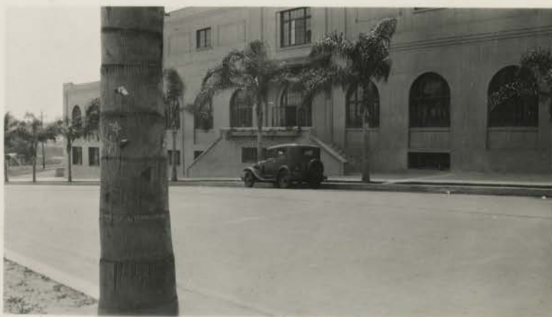
Main Building - Front Elevation
