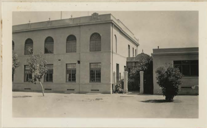
Main Building - Front Elevation
