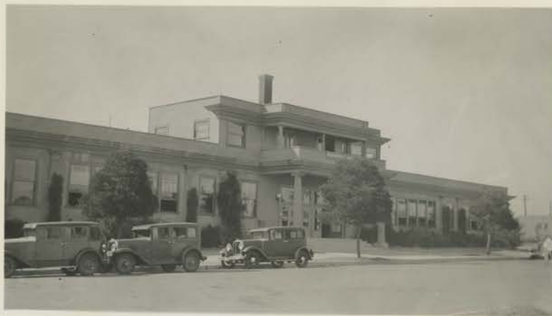
Main Building - Front Elevation of the Original Section.
