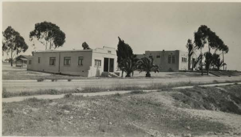
Auditorium Building - In Foreground Main Building in Background
