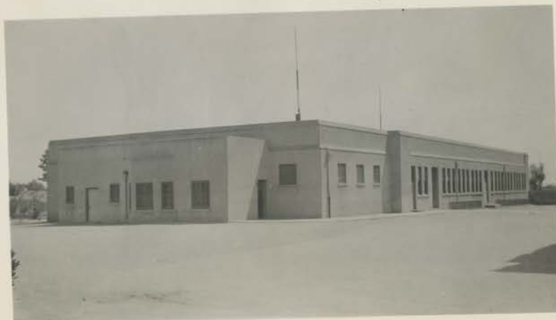
Building "C" - Northwest Corner
