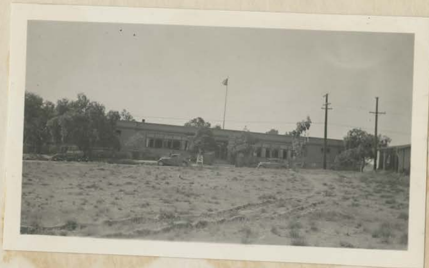
Main Building - Front Elevation
