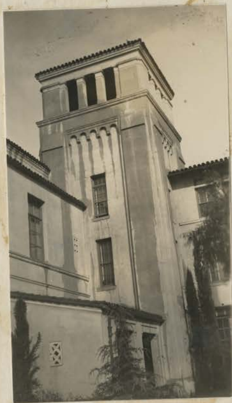
Main Building Front Elevation of the Tower.
