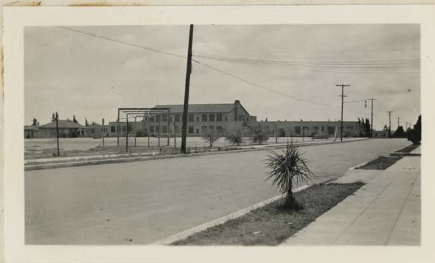
Main Building - Rear View Cafeteria Building at Left.
