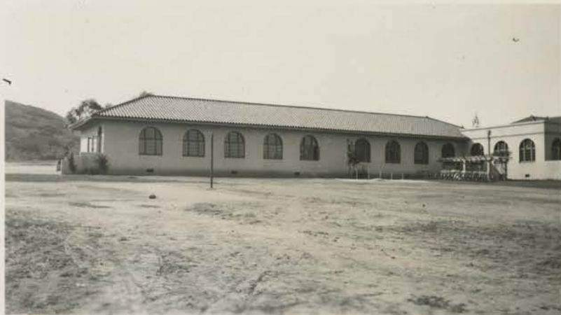
North Elevation of East Wing
