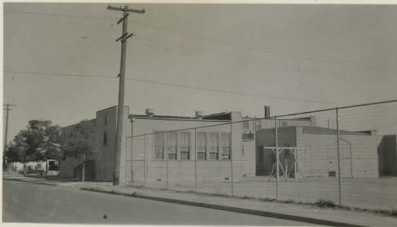
Main Building - Rear Elevation of Original Section
