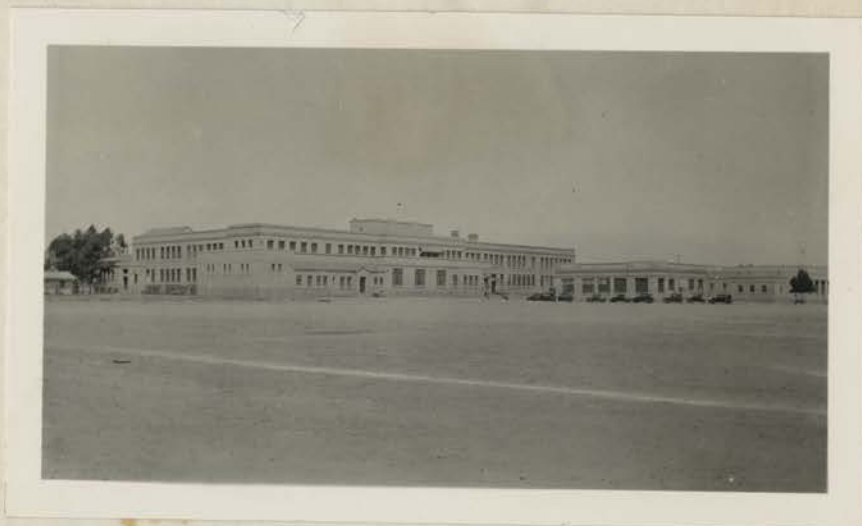
Main Building - Rear Elevation at left Manual Arts Building - Rear Elevation at Right
