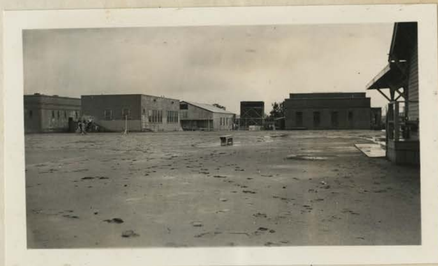
Auxiliary Buildings Boys' Shower and Locker Building at Left Temporary Building Center Girls' Shower and Locker Building at Right
