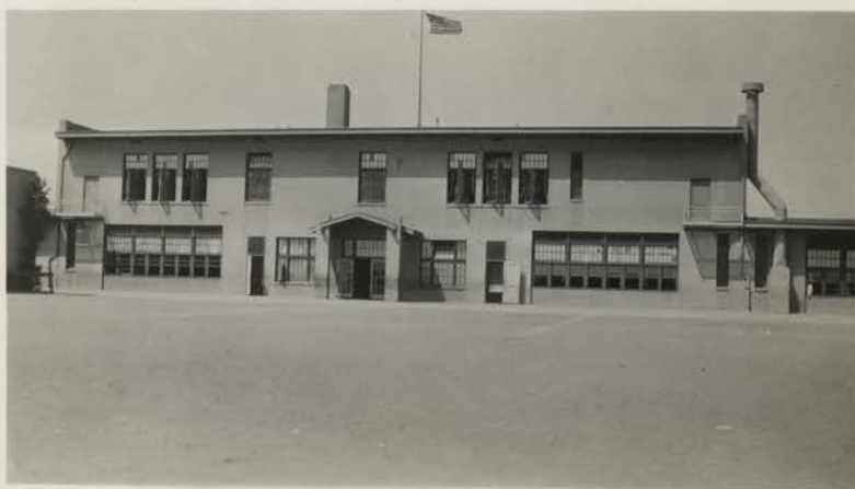
Main Building - Rear Elevation
