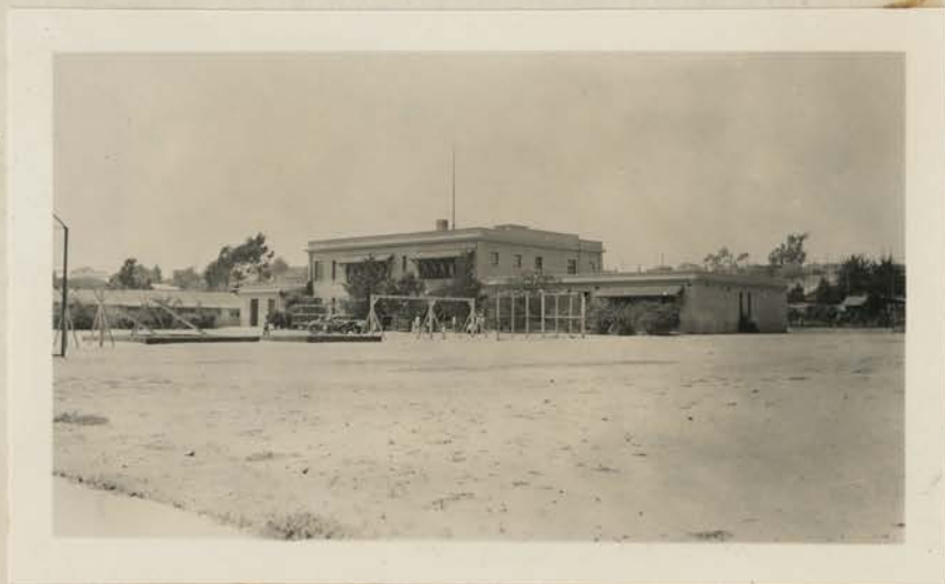
Main Building - Rear Elevation Temporary Buildings at Left.
