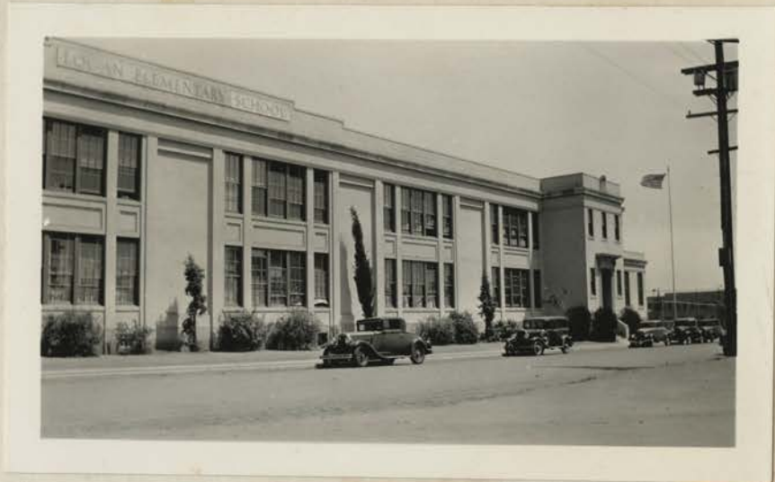
Main Building - Front Elevation
