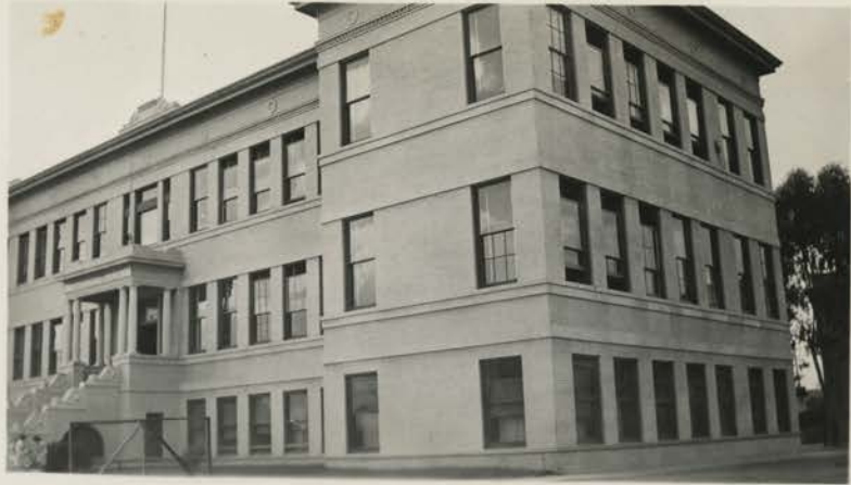
Main Building - Front Elevation
