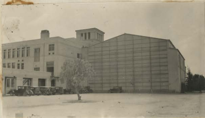
Main Building Rear Elevation Showing Temporary Rear wall at the Auditorium.
