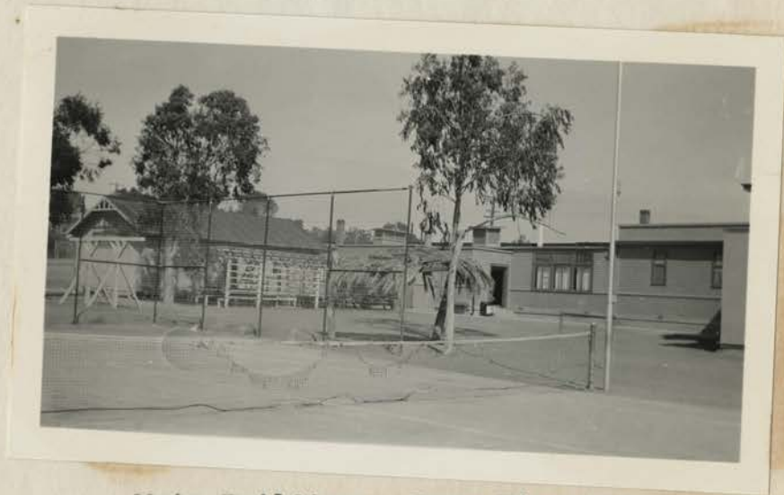
Main Building - Rear View and Elevation of Store Room Bungalow
