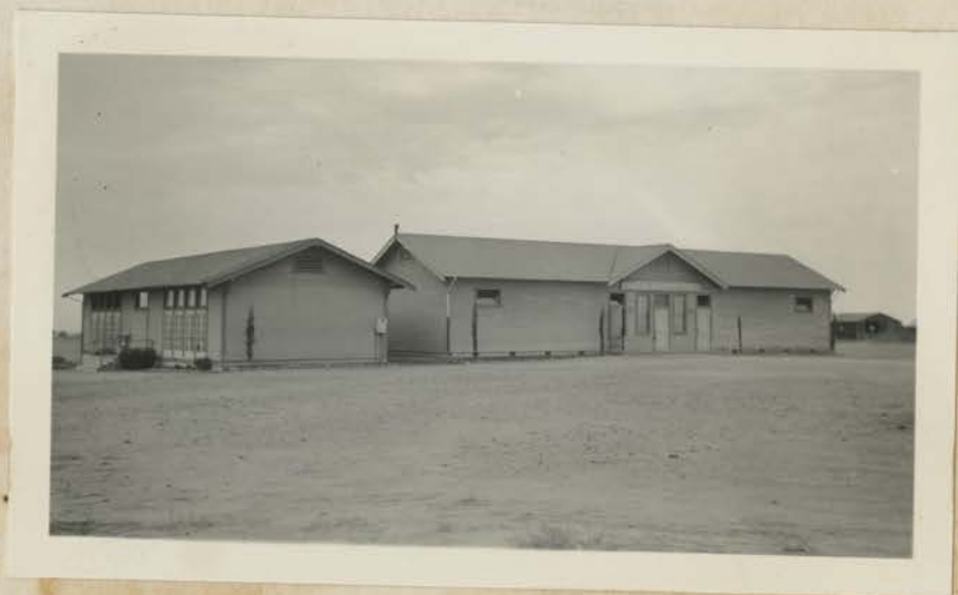
Rear Elevation of Main Building and Lavatory
