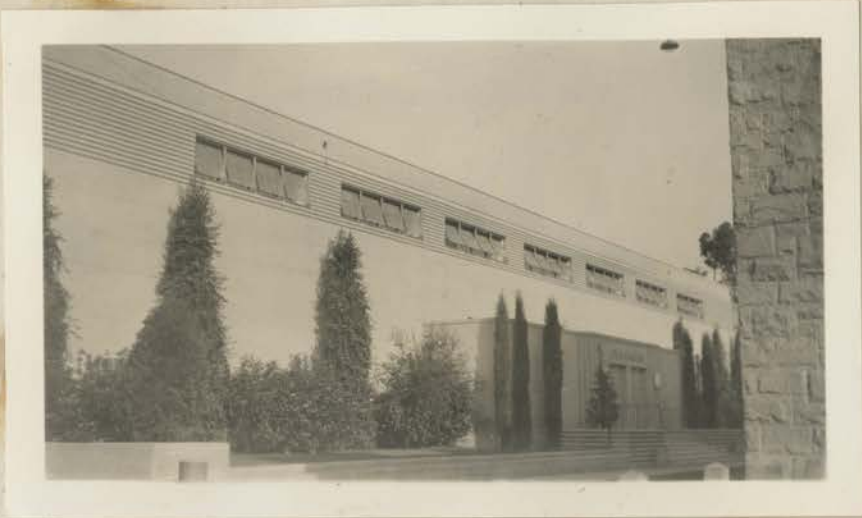
Gymnasium Building - South Elevation
