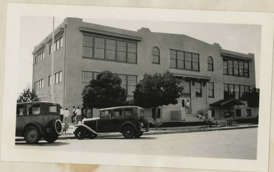
Main Building - Front Elevation
