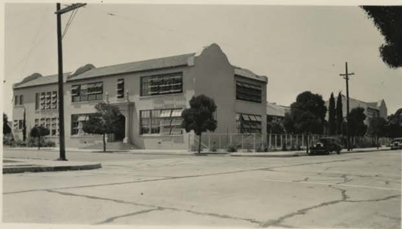
Main Building - End at Left, Front on the Right
