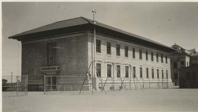
MAIN BUILDING - Rear Elevation
