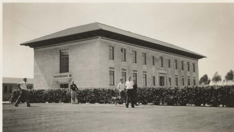
MAIN BUILDING - Front Elevation
