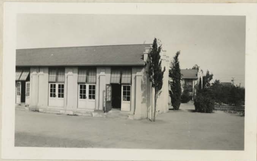
Main Building - Elevation of Southwest Corner
