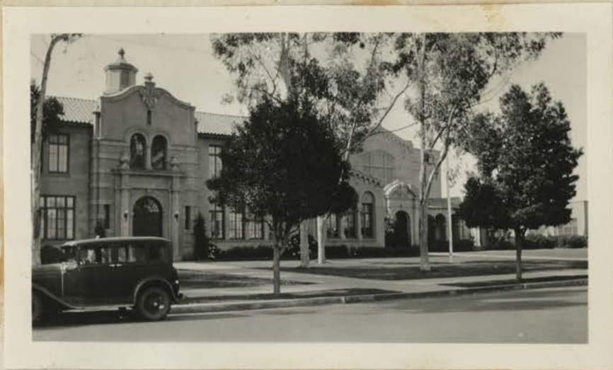
Main Building - Front Elevation in Foreground Auditorium Wing at the Right
