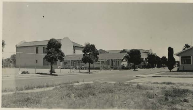
Main Building - End View and Rear Elevation Cafeteria Building in Foreground.
