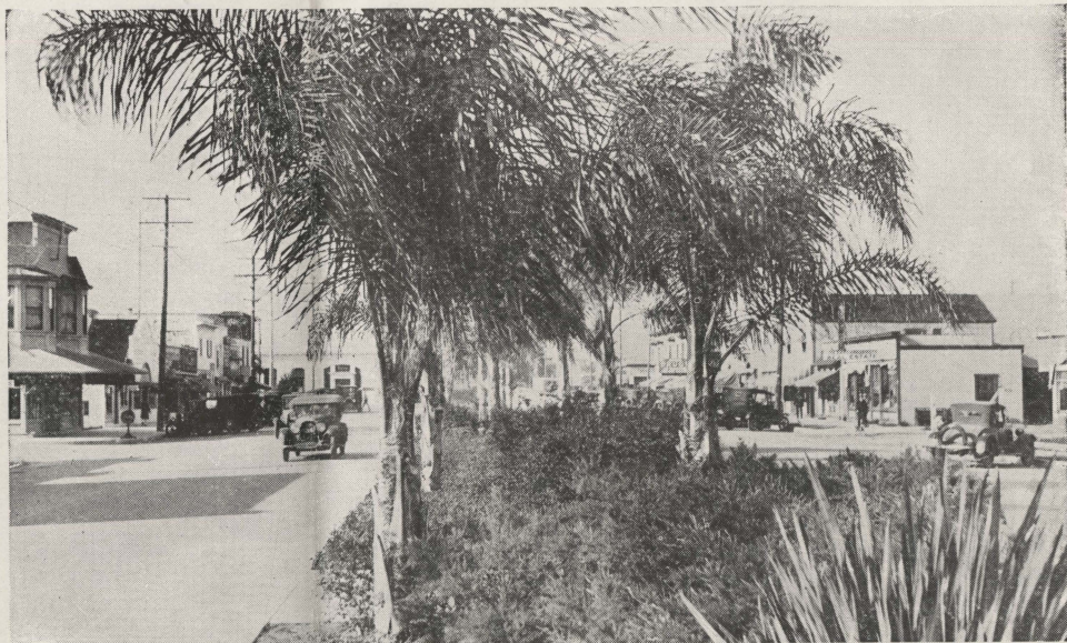
CHULA VISTA—WITH ITS BOULEVARD STREETS
