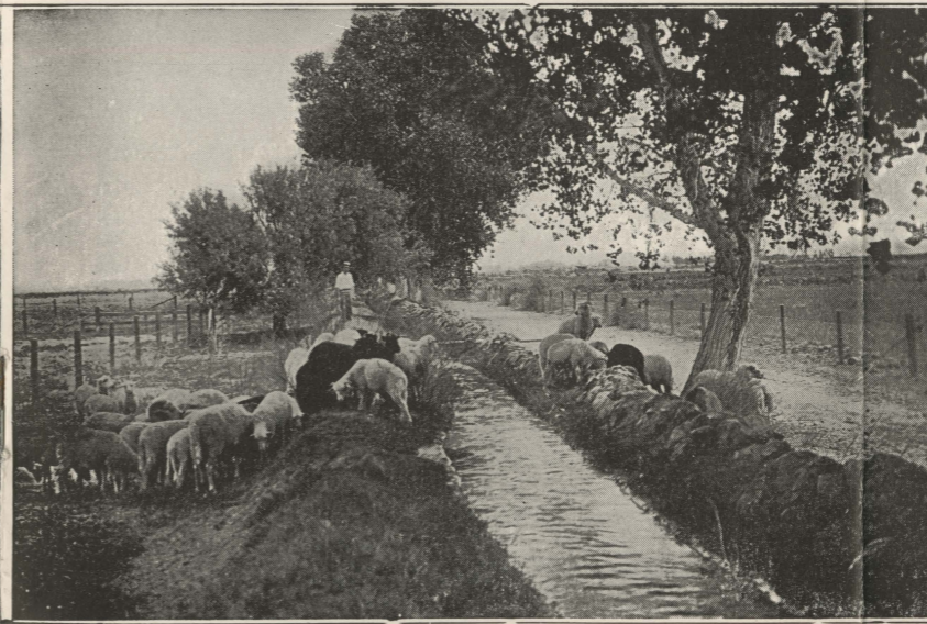
An Imperial Valley Irrigation Canal
