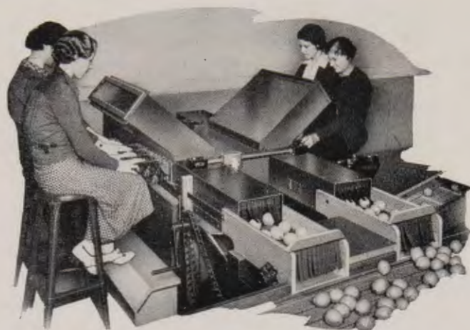
The Citrus X-Ray Machine developed with the assistance of the Exchange is credited with being the most important new development in the industry in recent years. This equipment permits accurate segregation of frost damaged fruit and of granulation in oranges and blossom-end decline in lemons, which are serious problems in some districts every season.
