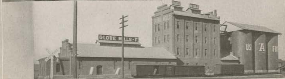
TYPE OF SAN DIEGO'S PASSENGER STEAMERS (UPPER)—TRAINLOAD OF CITRUS MATERIAL READY FOR SHIPMENT AT SAN DIEGO—ONE OF THE MANUFACTURING PLANTS OPERATING IN THIS SEABORD CITY—GLOBE MILLS WITH AN OUTPUT OF THOUSANDS OF BARRELS OF FLOUR ANNUALLY
