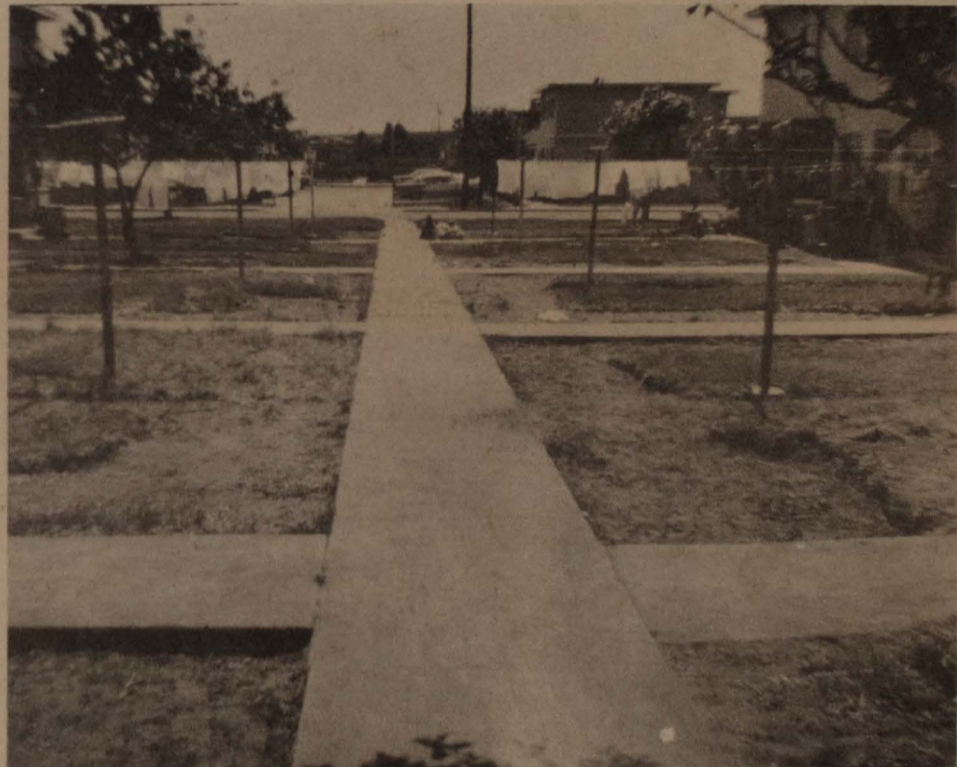
Oakland Housing Project without fences (Peralta)
